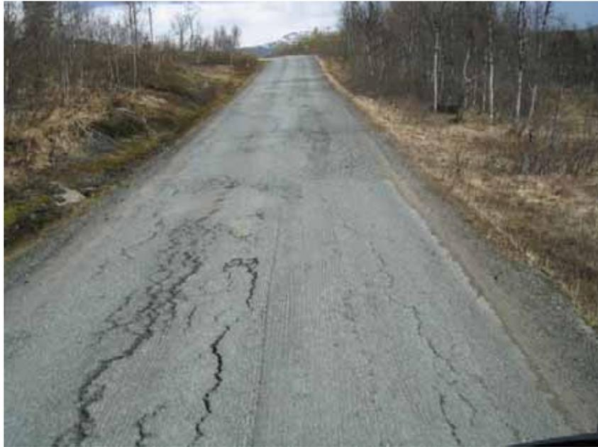
*Figure 2. A low volume road on the island of Senja in the Northern Norway suffering from permanent deformation problems caused by inadequate drainage and a too thin structure.*
