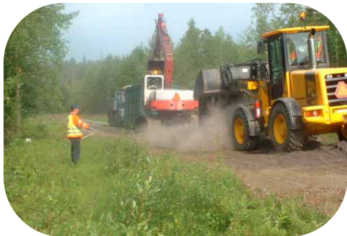
Spreading fly ash at road BD694, Vitåfors, Sweden
