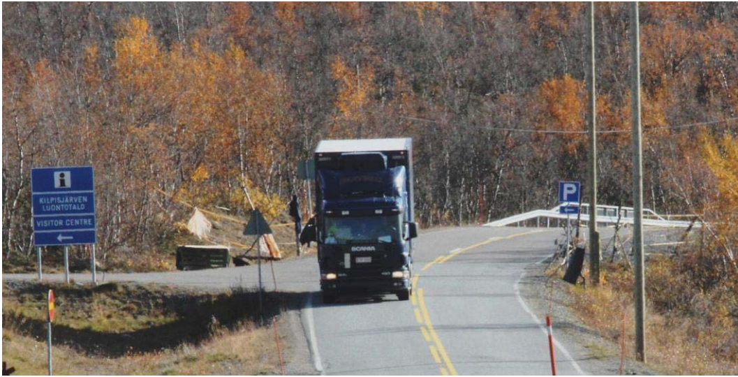
Figure 18 Test truck at an improperly banked outercurve on Highway 21 in Kilpisjärvi
