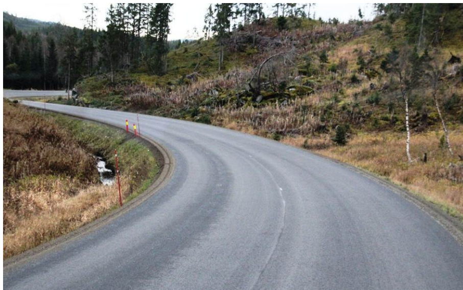
Figure 68 The Fjerdings S-curve is improperly banked after resurfacing 2011
