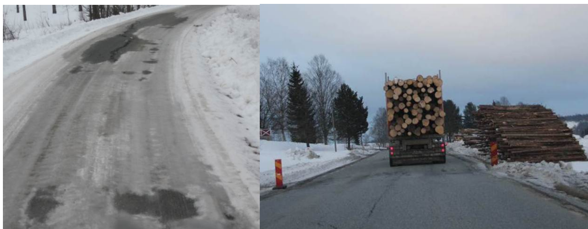
Figure 104 The winter conditions included driving on corrugated ice layers and uneven frost heaves
