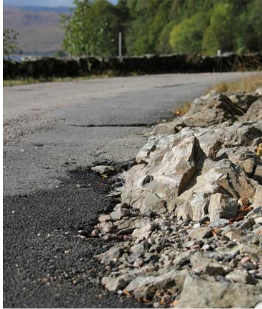
Figure 43 Hazardous rock edges at the pavement edge on Road B8005 at Loch Arkaig
