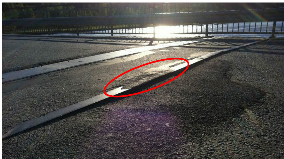
Figure 79 A very rough bridge joint at Nämforsen
