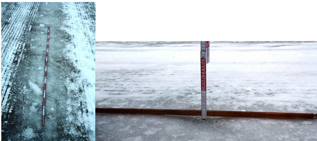
Figure 106 Remaining corrugations; note grooves created by the grader [Photo: J Granlund]
