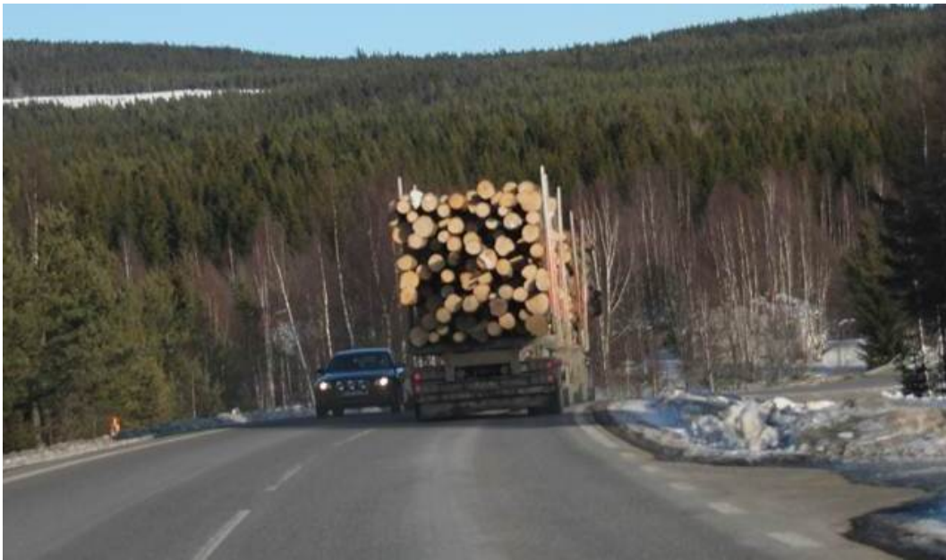
Figure 93 Unusual hazard: Insufficient crossfall of INNER -curve at Road 331 at Mo
