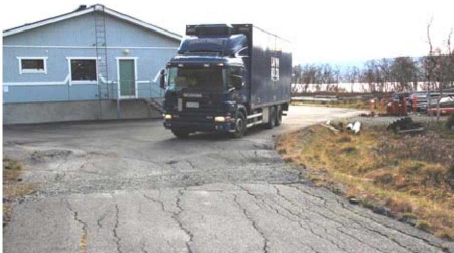
Figure 23 Road damages caused by frost action in the late winter season
