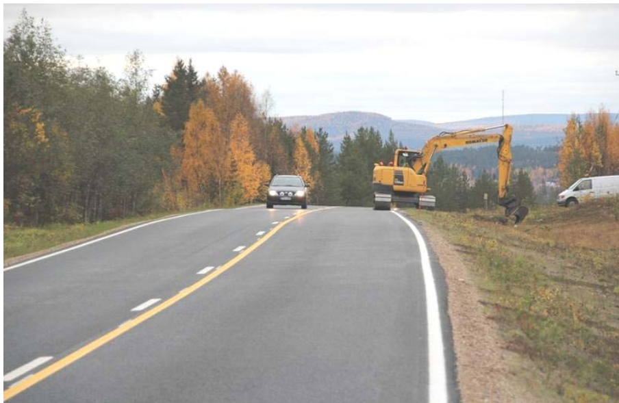
Figure 21 An excavator blocking part of the National Highway 21 without any warning signs
