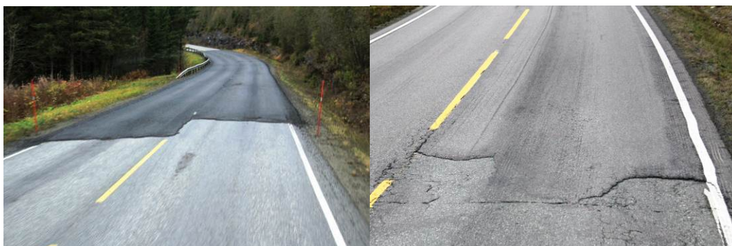
Figure 53 Improper transversal joints at new and old asphalt patch repairs on E6
