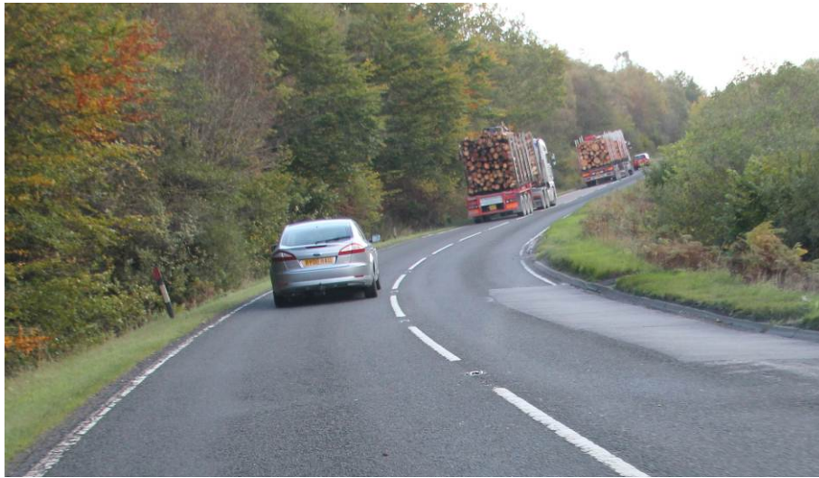
Figure 41 A82 has many improperly banked and thus hazardous sharp outer-curves
