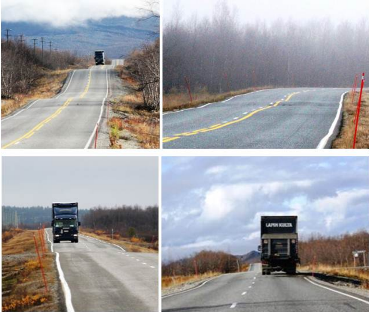
Figure 10 Thawing permafrost under Highway 21 gives severe settlements and a rough ride
