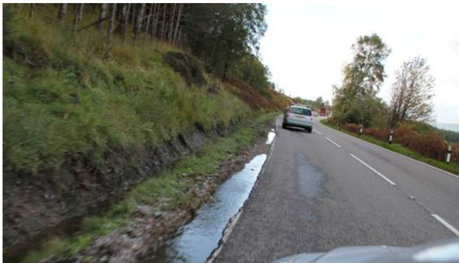
Figure 42 Water pooling in deformed shoulder at the exit of a sharp inner-curve on narrow A82
