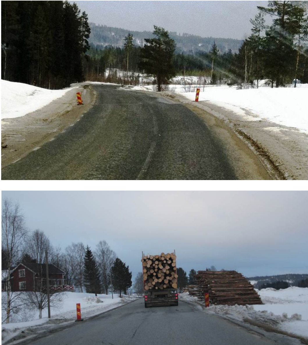
Figure 78 Roughness with several decimetre amplitudes, caused by frost action
