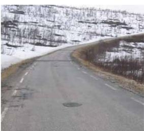
Figure 21. Road 232 in Senja was rated as a problem road in summer due to rutting, potholes and uneven frost heaves around culverts.
