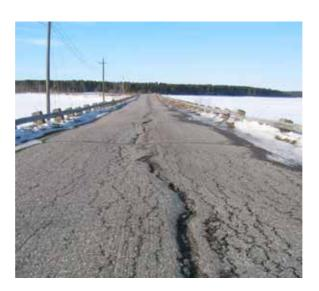
Figure 43. The narrow and poor quality road embankment section at Luusua on road 944 was reported to be a traffic safety hazard in the area. This section was repaired in summer 2003.
