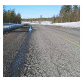
Figure 38. Road 19789 has severe deformation problems and sections with uneven frost heave.
