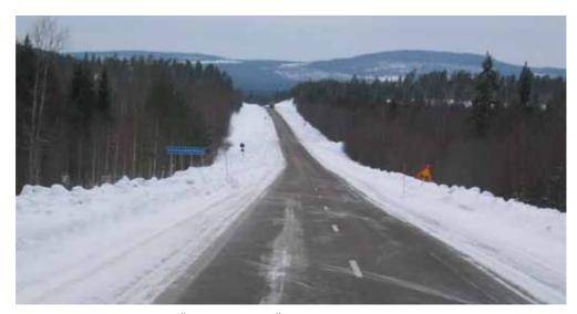
Figure 61. Road 98 between Övertorneå and Överkalix presents a good example of a road that is causing stress for heavy vehicle drivers. In this case a steep hill and an uneven frost heave "bump" in the bottom of the valley forces trucks to break - and if the road has ruts due to compacted snow or poor friction, drivers have problems controlling the vehicle.
