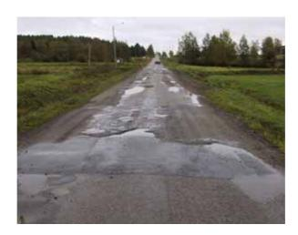
Figure 28. Rough and uneven roads were major problem for road users in Övertorneå – Överkalix. Road 915 is a good example of such a road. This road was also marked to be a road that respondents tried to avoid using (see chapter 7) and will be rehabilitated in summer 2004.
