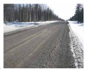
Figure 5. Road 19789 has been changed to a gravel road due to severe frost problems.
