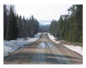
Figure 4. Road 855 is a typical gravel road in the Övertorneå area with spring thaw bearing capacity problems
