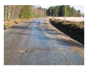
Figure 7. Road 3423 in Kuorevesi is a typical road with pavement damages on the inside edge of the curve.
