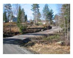
Figure 6. Gravel roads in Kuorevesi area are narrow and have problems with poor geometry, road 3424.
