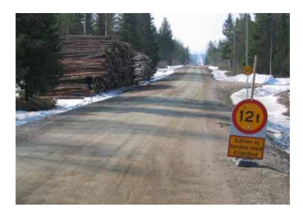
Figure 45. Due to load restrictions, road users complained about Road 855 in Övertorneå.
