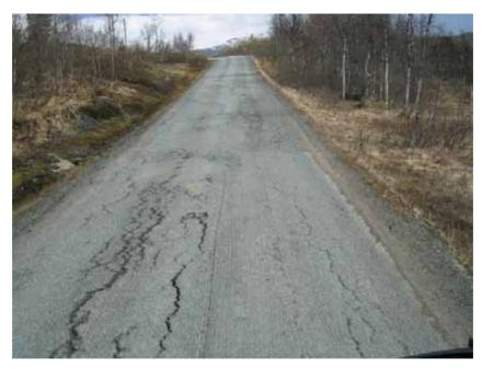
Figure 2. A low volume road on the island of Senja in the Northern Norway suffering from permanent deformation problems caused by inadequate drainage and a too thin structure.
