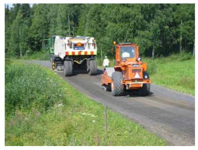
Figure 3. Improving the bearing capacity of the base course layer of a low volume road by means of stabilisation.
