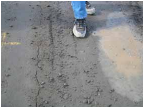
Figure 82. Cracking and water pumping in the wheel paths (left photo) and water pumping through a longitudinal frost crack in the road shoulder (left photo) after ten passes of a fully loaded maintenance vehicle.
