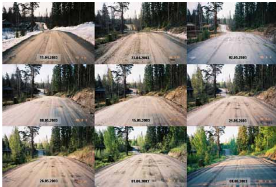
Figure 50. Photos from the Kuorevesi Percostation site during the spring thaw period in 2003.
