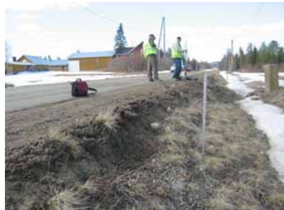
Figure 60. A 30 cm high vertical shear zone beside the right road shoulder at the Kemijärvi Percostation during spring 2004.
