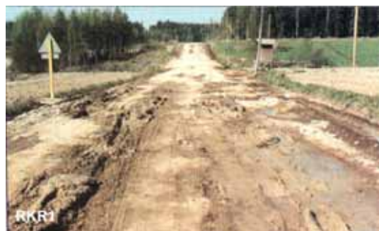
Figure 25. Example of Finnish spring thaw damage class 1 on gravel road (Painorajoitusohje 2004).
