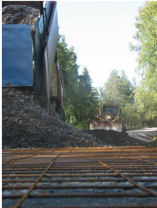
Figure 116. Base course is laid over steel grid. (photo: T. Ruohomäki)
