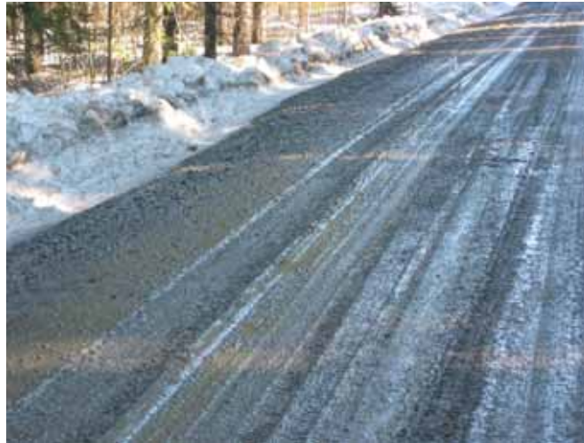
Figure 12. Early phase of surface thaw weakening on a gravel road. The frost level is only 40 – 60 mm from the road surface. (photo: S. Kohonen)
