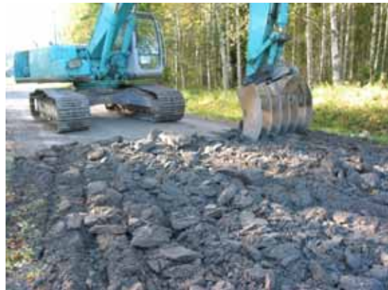
Figure 107. Homogenization of the top 200 mm of the structure. (photo: T. Ruohomäki)
