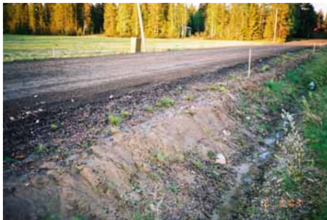
Figure 15. Plastic silt squeezing from the road shoulders during the structural thaw period at the Kemijärvi Percostation site in 03.06.2003.
