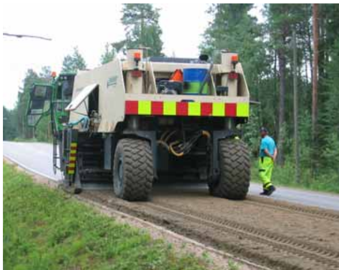
Figure 115. Homogenisation machinery made by Andament Oy from Finland. The same machinery can also be used for stabilization.
