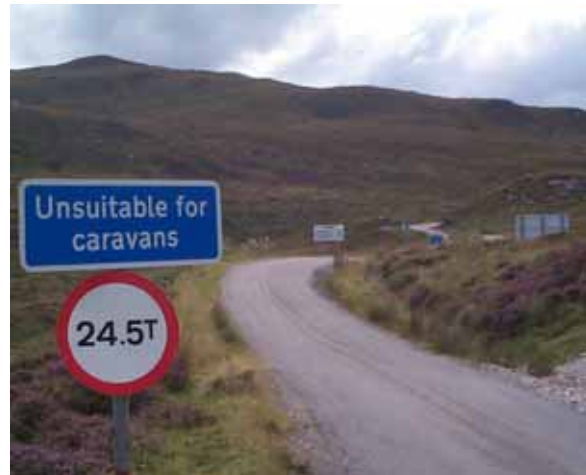
Figure 24. Road B869 Lochinver-Stoer-Drumbeg-Kylesku is a typical road subject to load restrictions in the Scottish Highlands. It is a 3m wide single track route with passing places that passes through some of the most rugged rocky scenery in the western Highlands. Its tortuous alignment makes it unsuitable for coaches or heavy vehicles over 24.5 tons.
