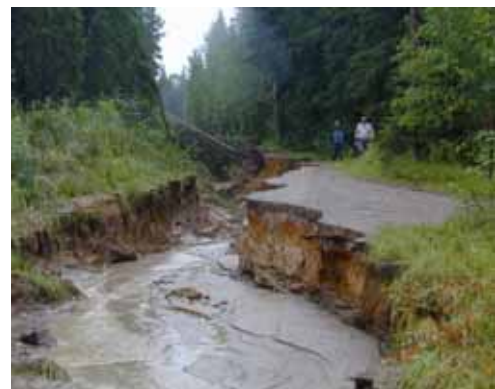
Figure 6. Heavy rains can cause major erosion problems on low volume roads if the drainage system is not working well enough.
