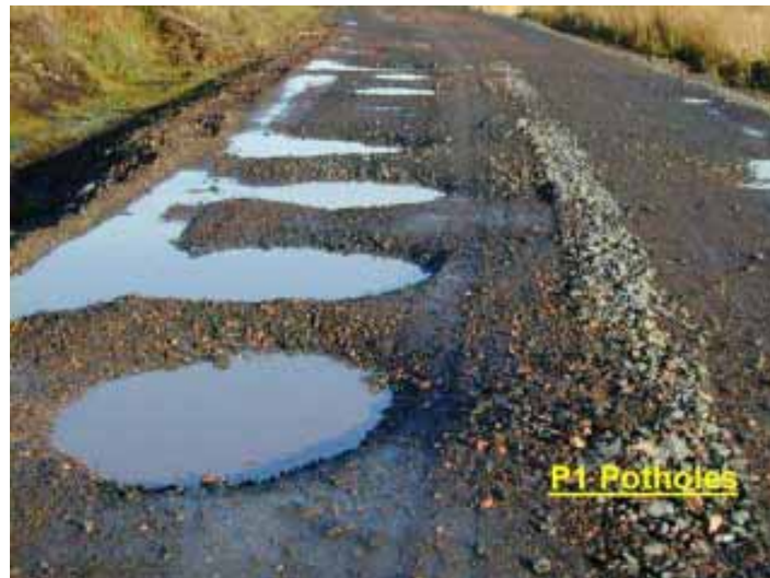
Figure 14. Example of class P1 deep potholes according to the Scottish forest road intervention level description (Forestry Commission 2005).
