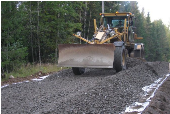
Rehabilitation of road on peat Extra load = additional settlement
