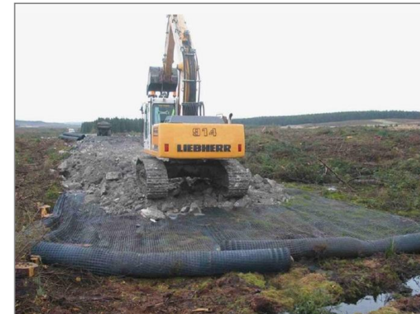
Low volume wind farm road immediate loading by 150 tonne trucks
