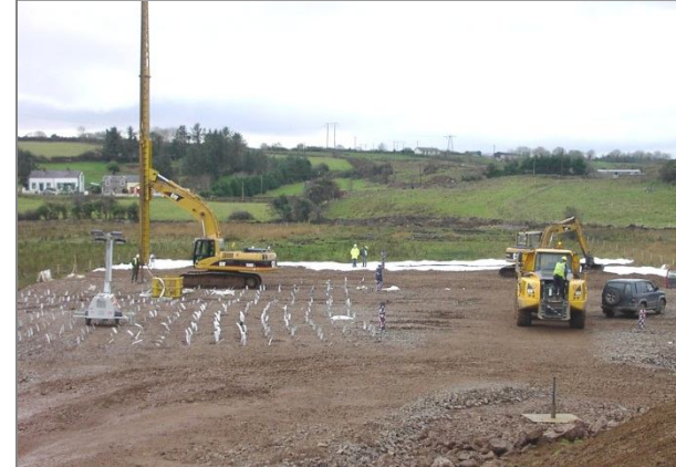
Vertical drainage to speed settlement – add €€€€€
