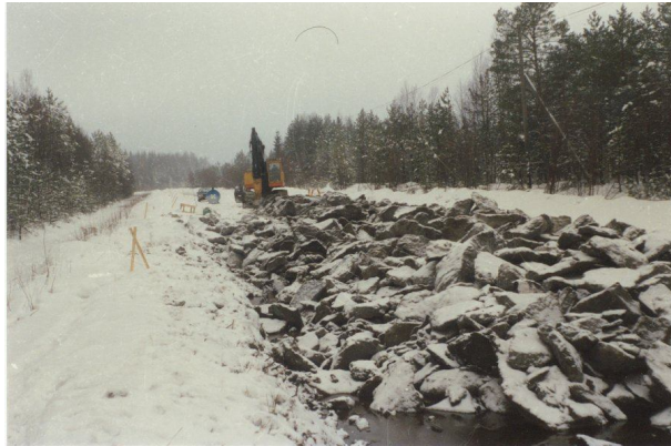
Work planning - excavation in winter when the peat is frozen
