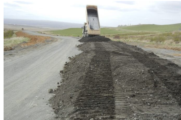
Widening of road on peat How to make the new act like the old
