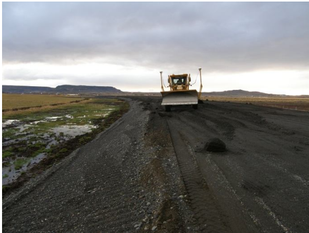
2-lane road in Iceland constructed by preloading – 1 year
