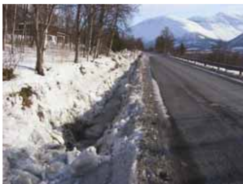
Figure 3.3. Removal of ice and snow from the ditch.
