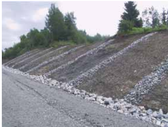
Figure 3.10. An example of making road cut slope more stable.
