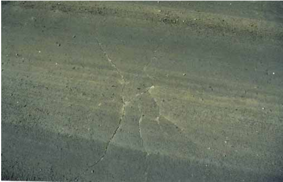
8b) Cracking, severe
