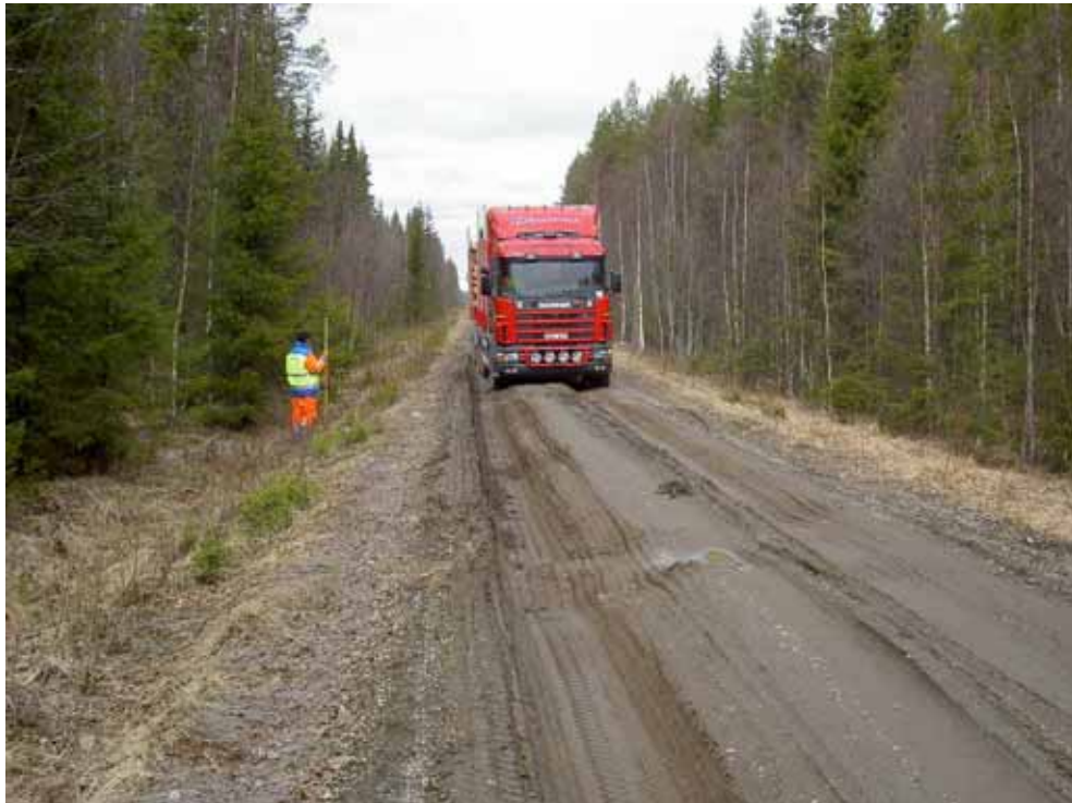
5b) Rutting, severe
