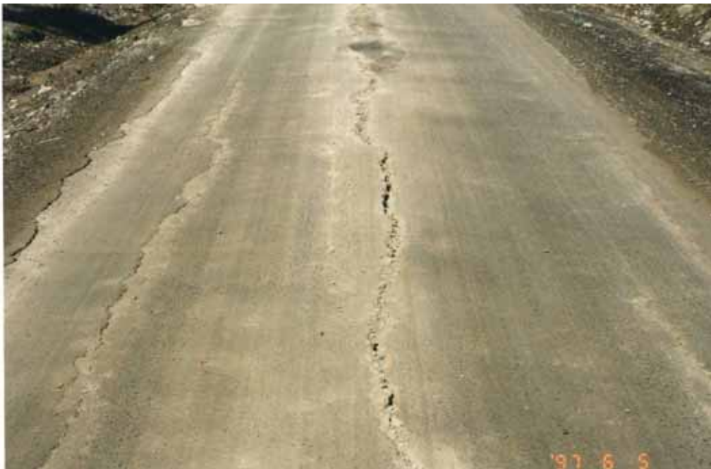
8b) Cracking, severe
