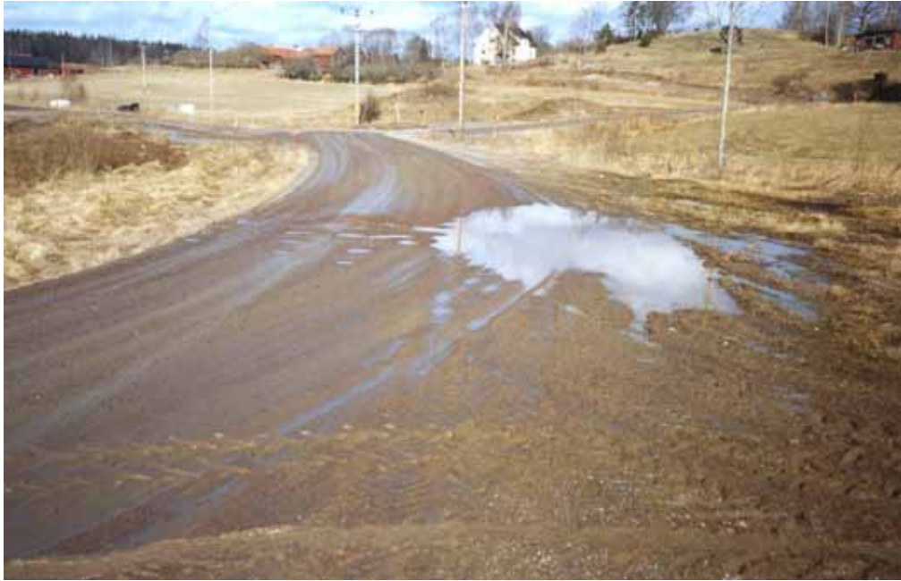
9b) Standing water on the road surface, severe
