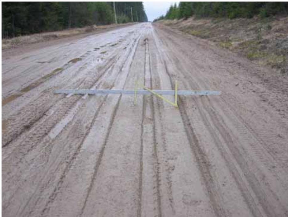
7b) Surface softening, severe
