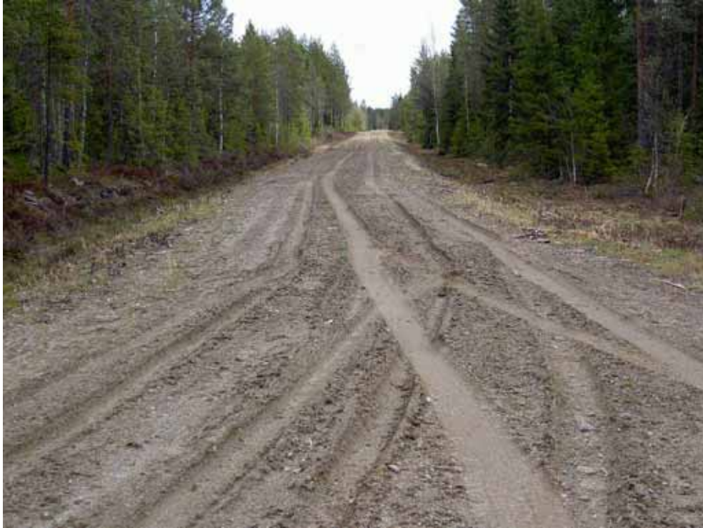
5b) Rutting, severe
