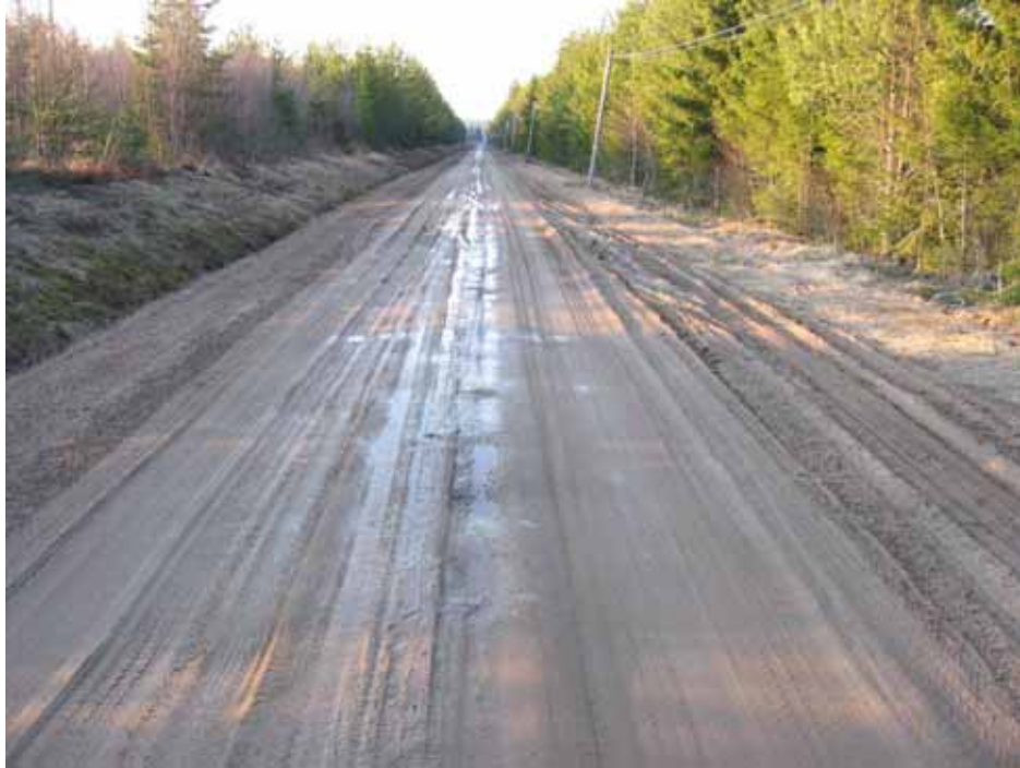
7b) Surface softening, severe
