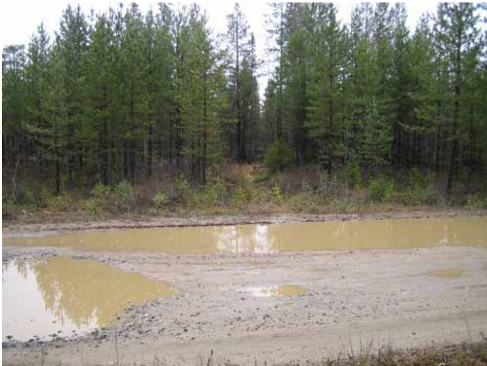
9b) Standing water on the road surface, severe
