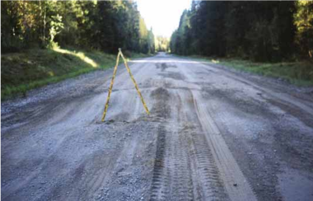
6a) Frost damages, minor
