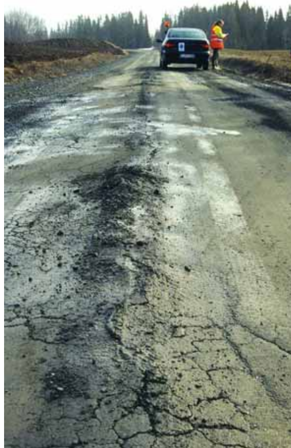
6b) Frost damages, severe
