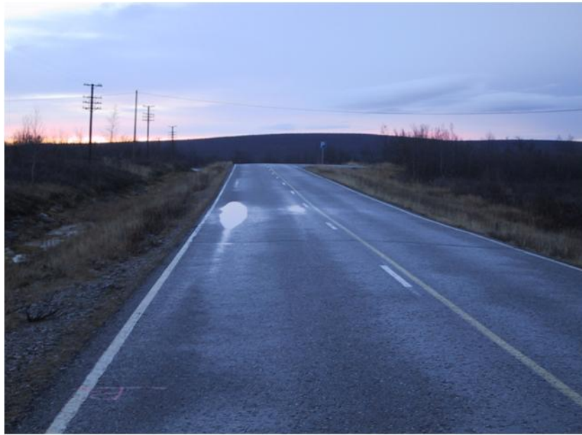
Figure 2.5.1. Poor drainage causing edge deformation in a widened section of Hw 21 in Kilpisjärvi, Finland. Note the standing water in the ditch at the same location as the worst deformation.
