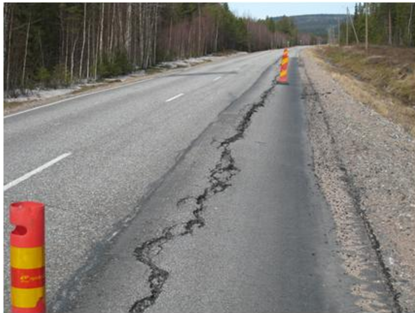
Figure 2.4.1. Differential frost heave between an old and an widened road section on road 934, an example from Finland.
