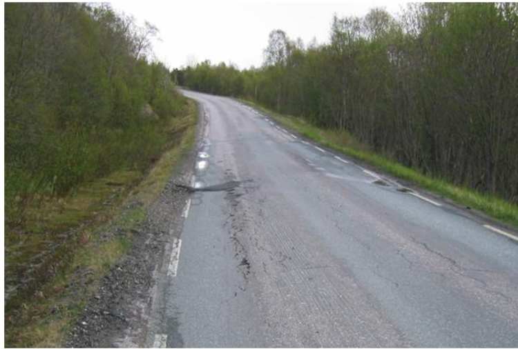
Figure 2.6.2. Edge deformation caused by a steep inner slope combined with poor drainage, an example from Norway.
