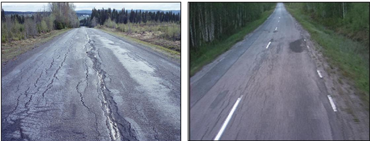
Figure 2.4.4. Examples of paved roads with widening problems due to Mode 2 rutting, examples from Sweden
