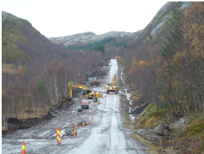
Figure 4.11.1. The important thing in road widening project is to ensure that traffic can use the road during the construction. An example from a road widening project in Norway.
