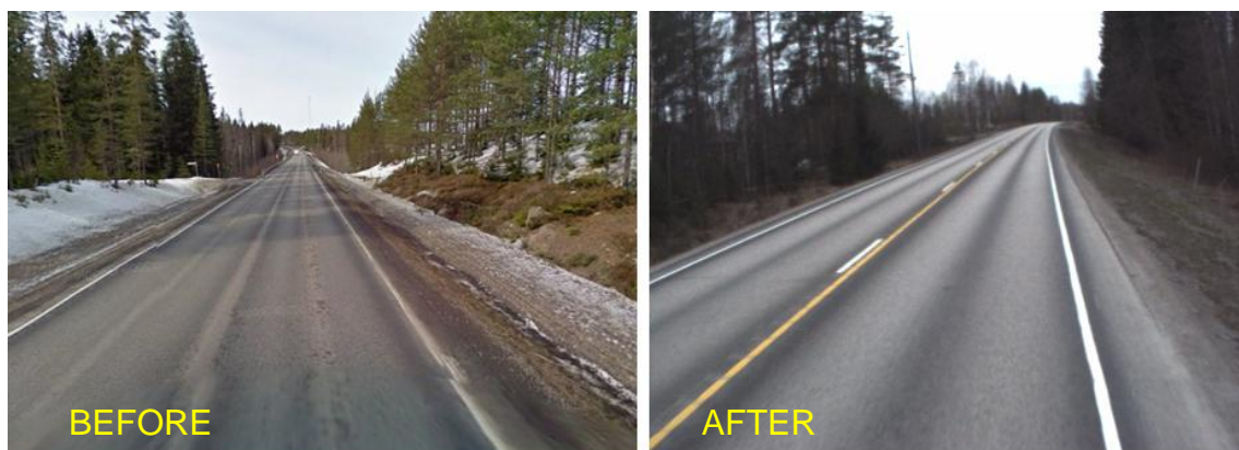
Figure 4.8.2. Widening to both sides on HW9 in Suonenjoki, Finland. After widening the traffic load is still on the old lanes and the widening is for the shoulder and safety area only.
