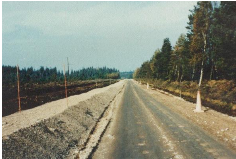
Figure 4.5.3. Widening of a floating road over peat by preloading
