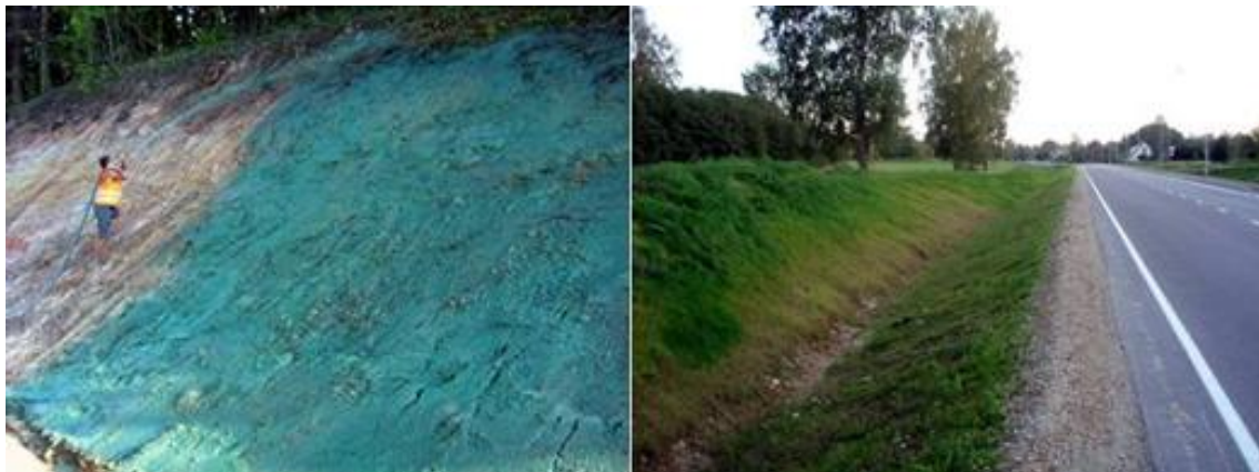
Figure 4.6.3. An example of a slope support solution using hydraulic seeding
