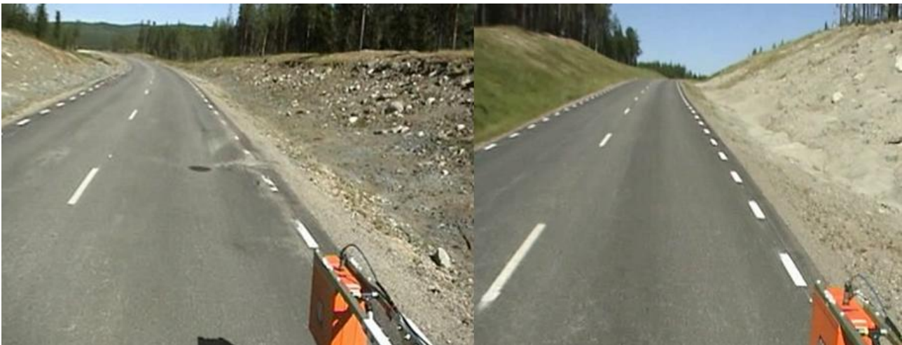
Figure 2.6.1. Poor outer slope stability causing problems for road performance, examples from Sweden.
