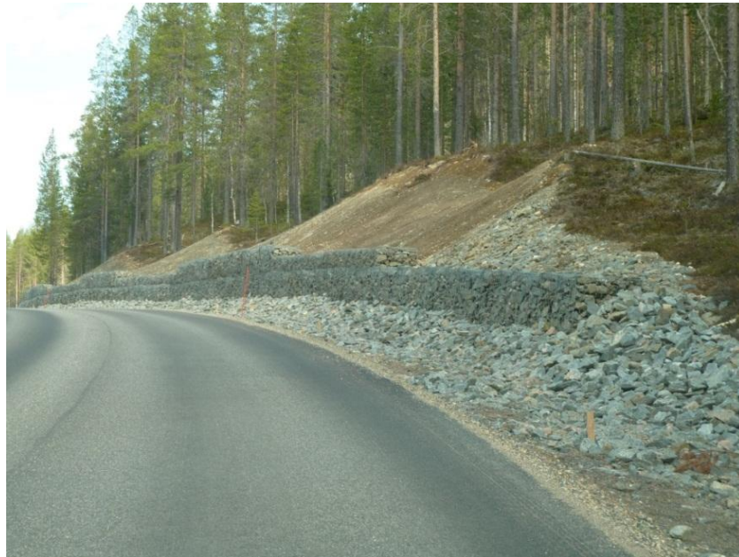
Figure 4.6.2. An example of a high quality slope support and drainage solution using gabions and heavy rip-rap in a problematic section with lack of space and side sloping ground
