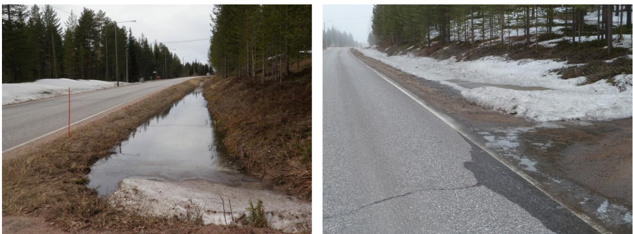
Figure 42_1. An example of a clogged private access road culvert from road 934, section 3, right ditch. Photographs are taken in spring 2010 (left) and in spring 2011 (right). The private road access culvert (chainage 1700 m) was frozen in both years and water was flooding into the ditch and flowing to the road.
