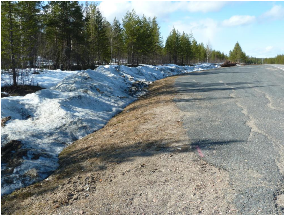
Figure 42_6. An example from highway 21, section 151, chainage 2000m. Melting snow behind the rest area keeps the ditch wet and prevents the flow of water. This has caused damages to the rest area and to the main road.
