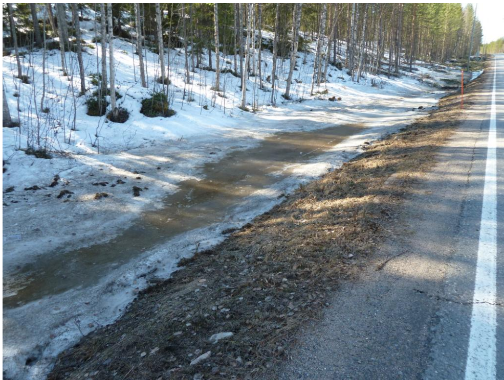
Figure 42_3. Sheet ice on road 926, at the beginning of section 19. The road is on side sloping ground and water is flowing from the slope creating sheet ice. Shoulder deformation, alligator cracking and transfer cracking were observed on this road.
