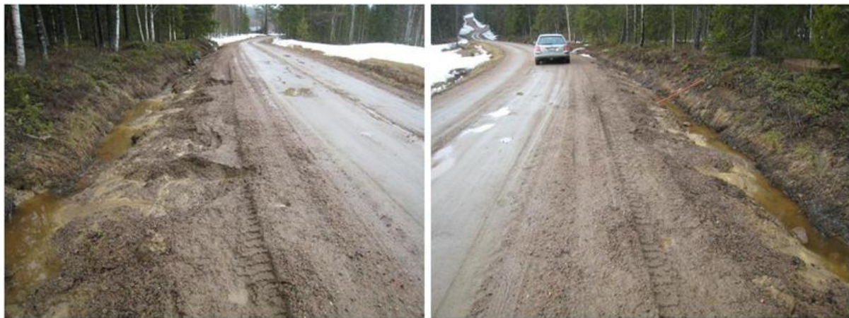
Figure 432_8. Clogged side ditch causing road problems and frost heaves on the local road 19686.
