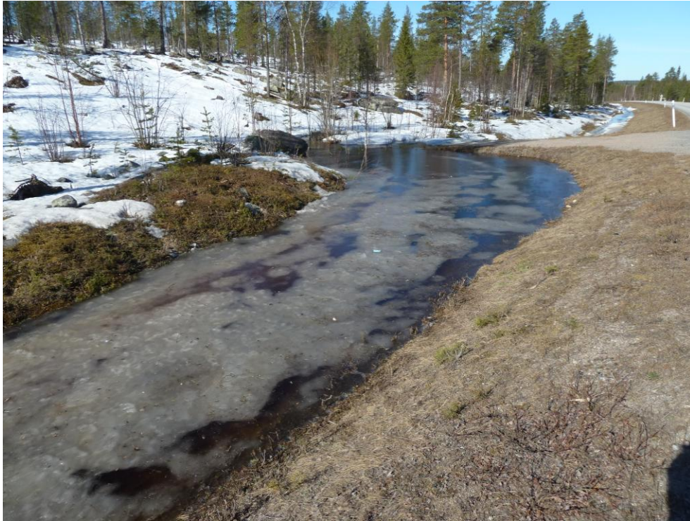
Figure 42_2. An example from road 78, section 219, left ditch, from spring 2011. At chainage 8030m the private road access blocks the water flow and creates a pond in the ditch causing water to infiltrate into the road structure.
