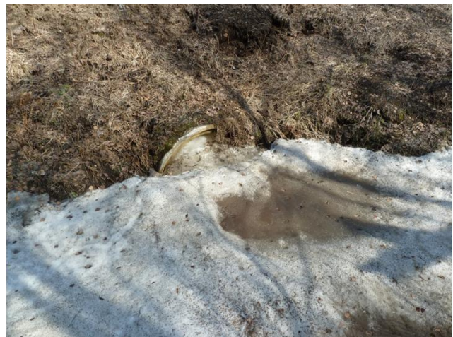
Figure 42_5. An example from road 80, section 12, from spring 2011. The left ditch is flooding (chainage 4590 m forward), because the main road culvert (chainage 4960 m) is frozen and stopping the flow of water from the left ditch to the outlet ditch.
