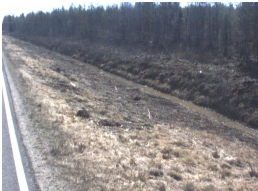
Figure 432_4. Ditch in adequate condition. The ditch has water as the longitudinal gradient is not sufficient in the left ditch. An example from road 926, section 17, chainage 5300 m.
