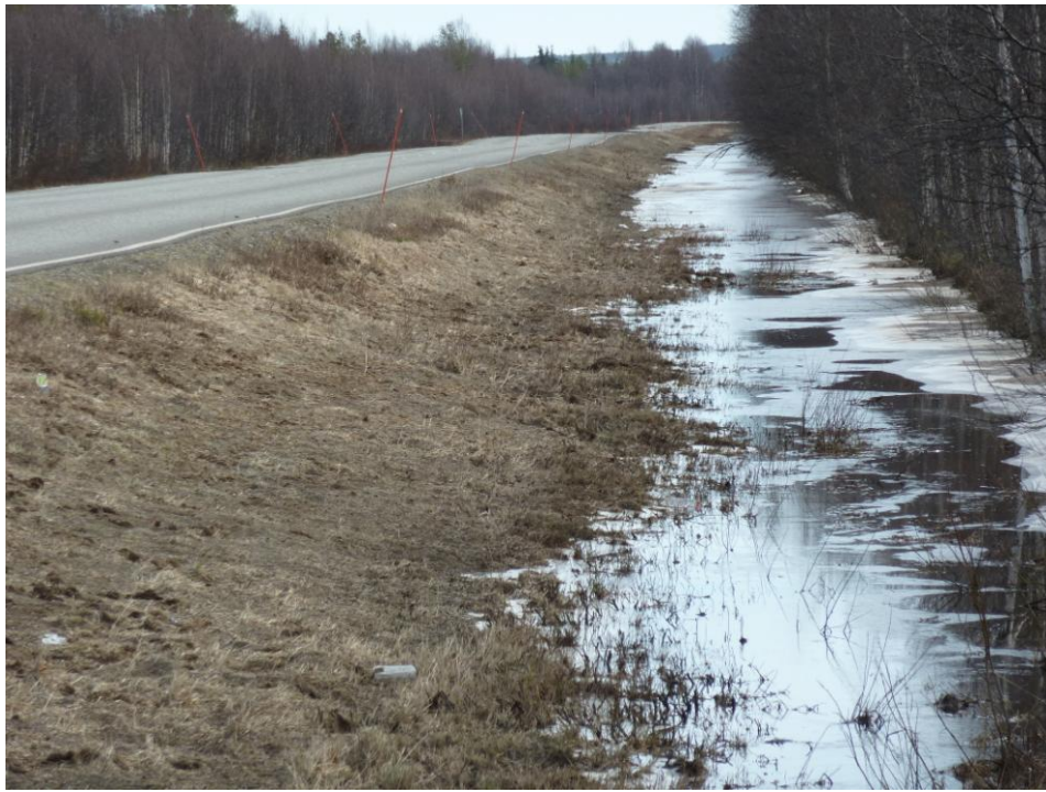
Figure 42_4. An example from road 80, section 11, from chainage 3980 m forward. The side ditch is full of water and there are frost heaves on the road.
