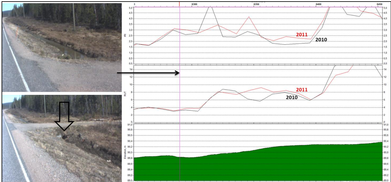
Figure 432_7. Example from road 934, section 3. The private road access culvert (chainage 6290 m) has been poorly installed (and clogged) and is blocking the water flow. The rutting values (second frame on the right) are high at the private road access, and rise even higher further on. Water above the clogged culvert is saturating the soil in the ditch slopes and the high water table is causing the growth of rutting and roughness values. The IRI values are shown in the upper right.
