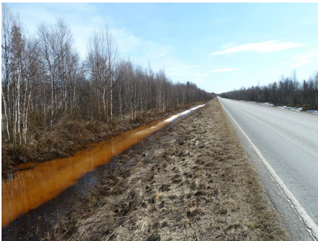
Figure 42_5. An example from road 80, section 12, from spring 2011. The left ditch is flooding (chainage 4590 m forward), because the main road culvert (chainage 4960 m) is frozen and stopping the flow of water from the left ditch to the outlet ditch.
