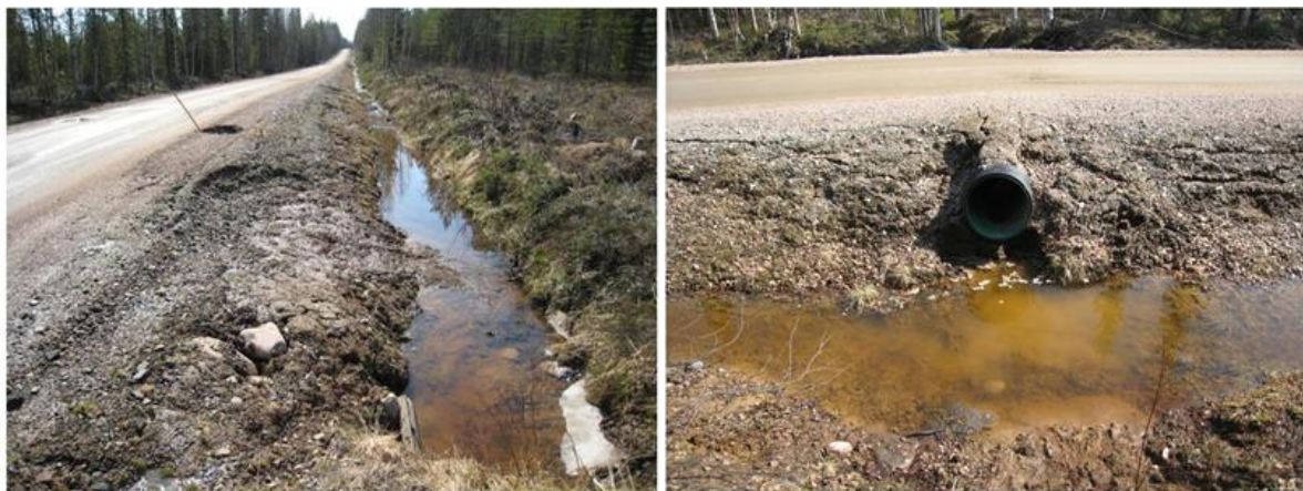
Figure 432_9. A clogged private road access culvert has caused the water level in the ditch to rise and soil flow from the inner ditch slope (left). The stick in the road shows the location of a big hole in the road due to melting ice lens (left photograph). The right photograph shows an example of a poorly installed main road culvert. Both examples are from road 19688.
