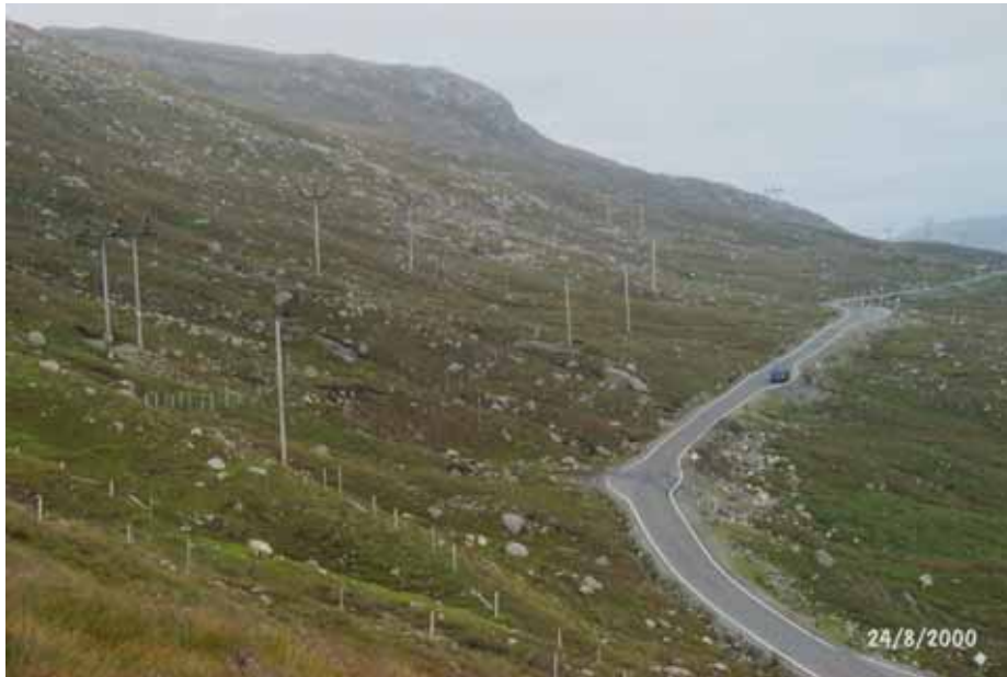
Figure 4.4. Single-track lifeline road in the Western Isles (photo Ralph Shackleton, The Western Isles Council).
