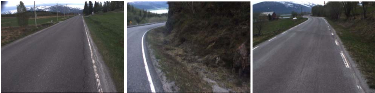
Figure 7: Examples of road sections with drainage Class 2 in Region Nord in Norway.
