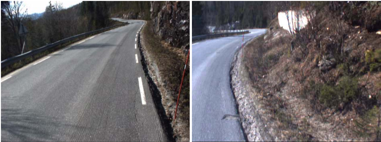
Figure 59: Erosion damages on the edge of the pavement, chainage left: 7650m, right: 8700m.
