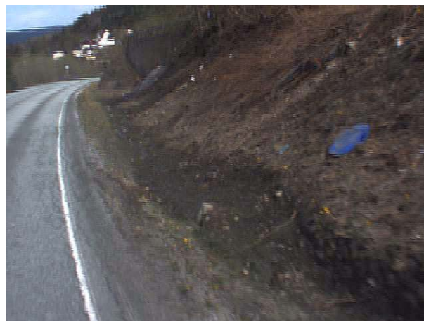
Figure 35: Partly blocked ditch on the upper side of the slope at chainage 5320m.
