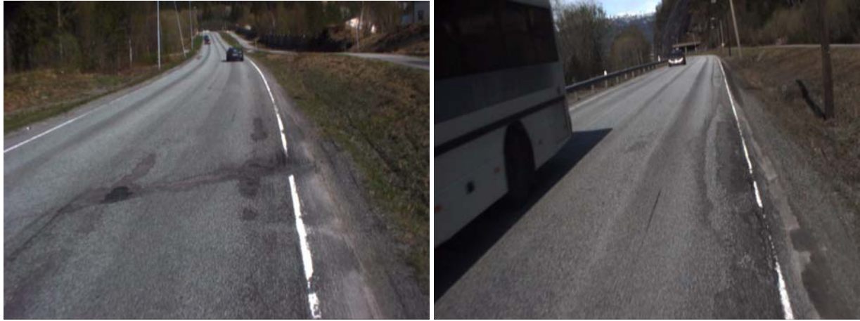
Figure 36: Road damages because there is little room for ditches, chainage left: 1160m, right: 2110m
