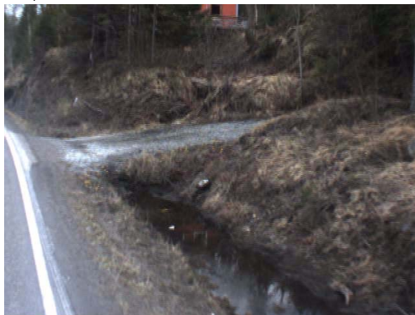
Figure 33: Private access road junction is blocking the water at chainage 4160m,
