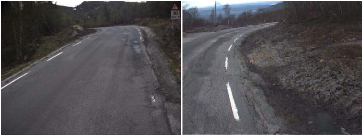
Figure 49: Drainage deficiencies (left: 13950m, right: 16740m).
