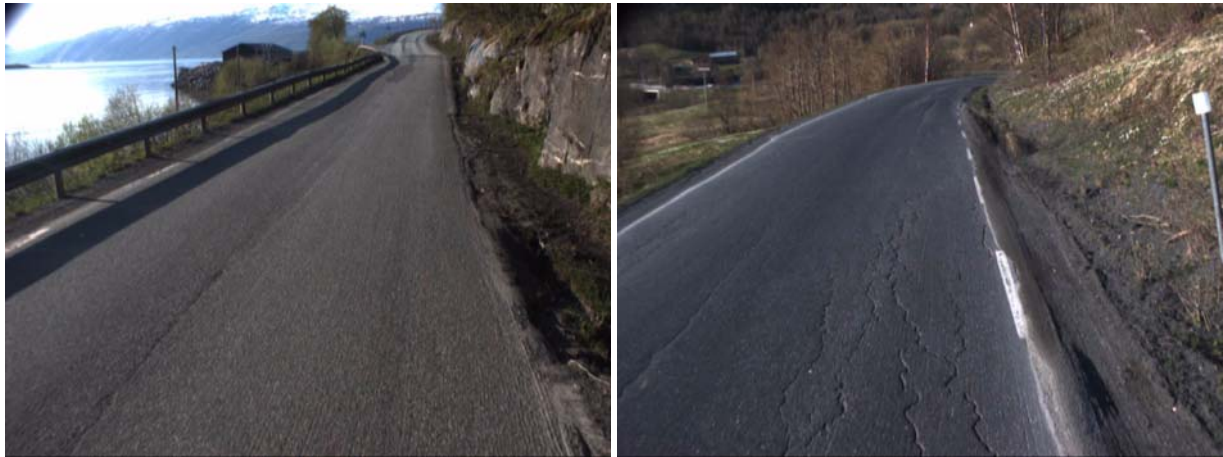
Figure 54: No room for a decent ditch, chainage left: 2690m, right: 11500m.
