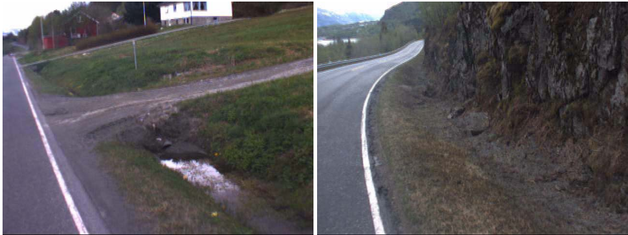
Figure 45: Left: Clogged culvert at chainage 4040m, Right: High verge at 11700m.
