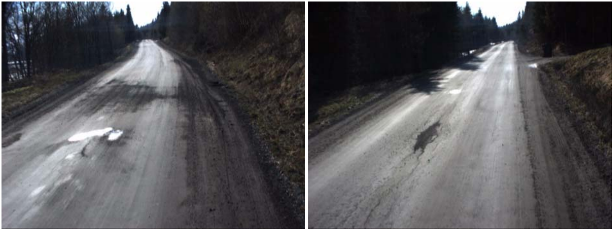
Figure 67: Drainage deficiencies on the upper side of the slope (Chainage 1330m and 1440m). Poor drainage is also causing Mode 2 deformations on the road, which can be seen as cracks in the road centre.
