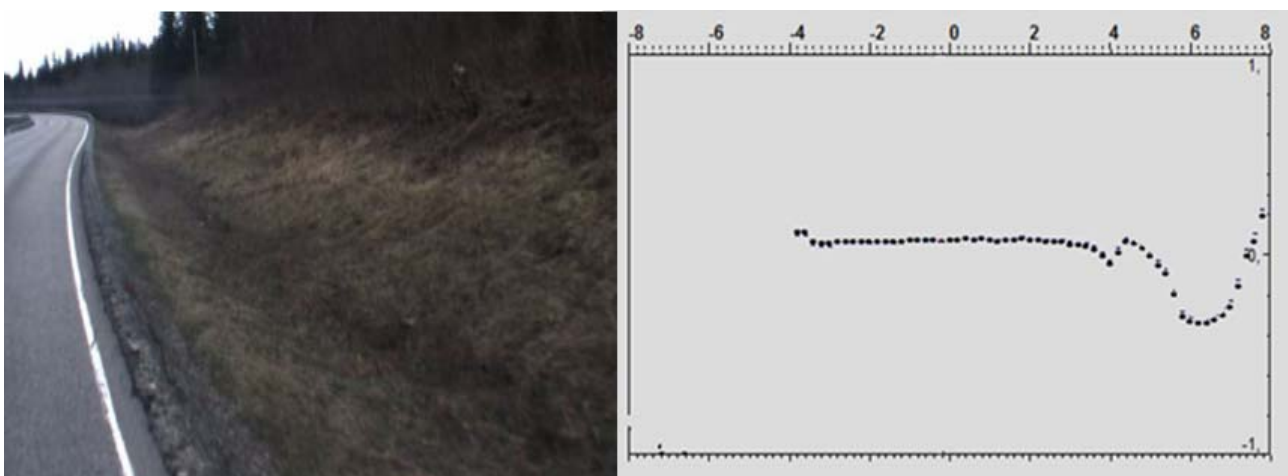
Figures 27: Inner slopes of road have lost their shape and verges have been formed. The ditch depth is only 50cm, example at 5160m. Erosion can also be seen at the pavement edge.
