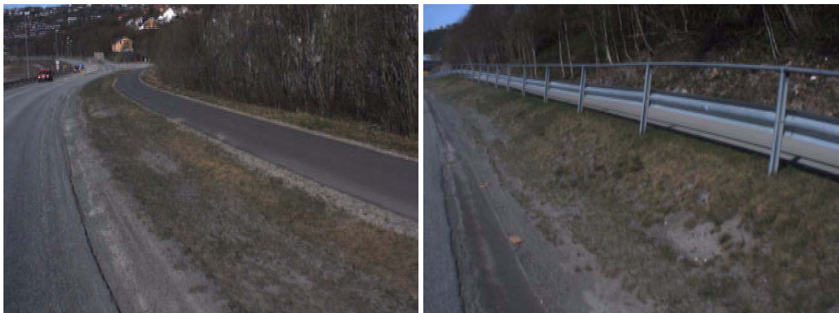
Figure 23: No drainage system between the cycle path and the E6 road (chainage 5445m, 5910m)
