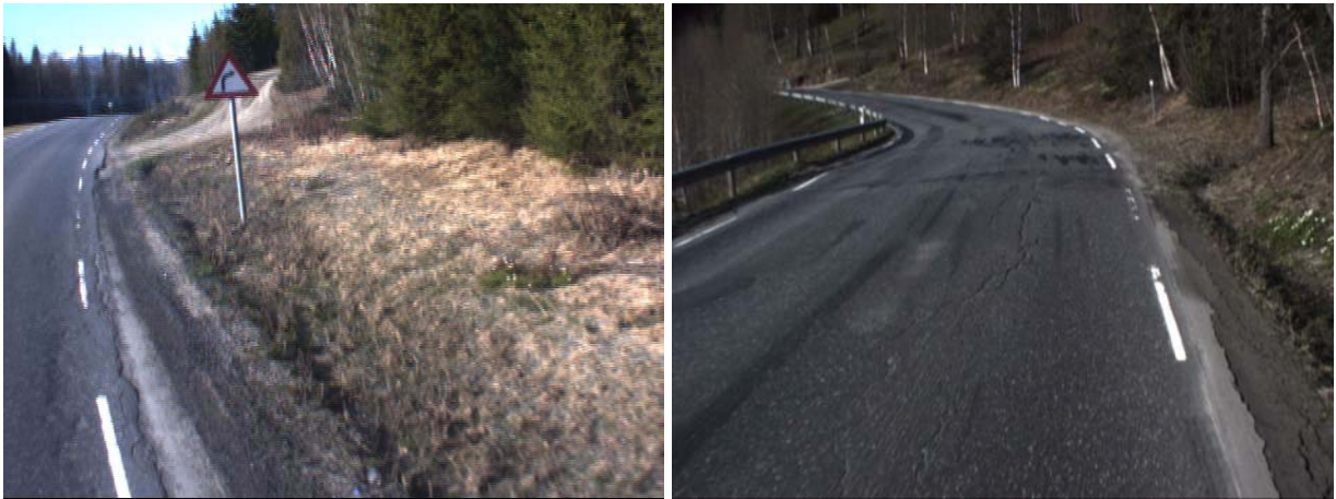
Figure 14: Drainage problems in a steep side sloping road profile, chainage left: 4530m, right: 4960m
