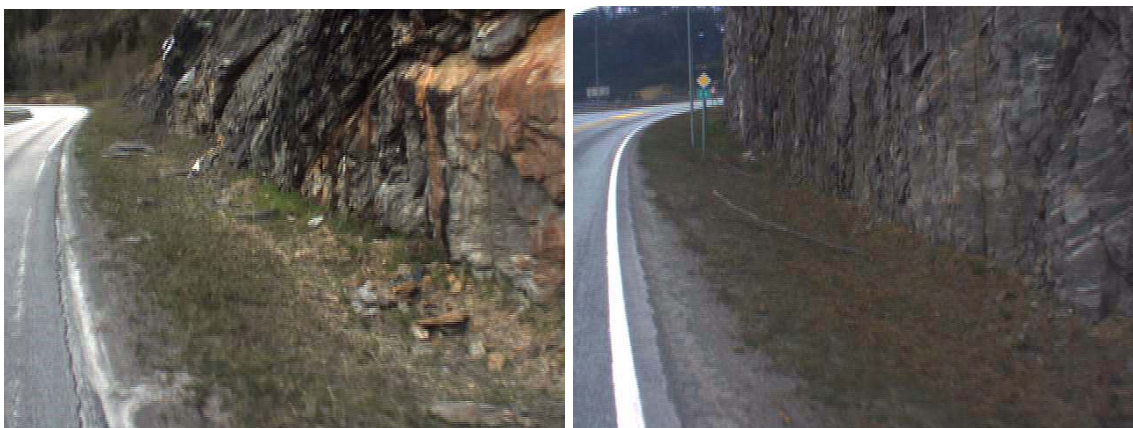
Figures 28: Left: Stones in the bottom of the ditch at chainage 2180m. Right: Rock cutting with good ditch depth at 3500m.
