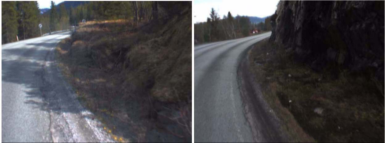
Figure 29: Examples of erosion, Left: Shallow ditch filled with unstable material at chainage 5530. Unstable material has filled the ditch at 8560m.
