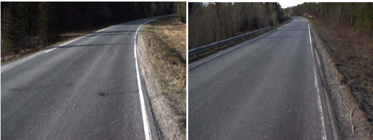
Figure 21: Verge is blocking the water, chainage left: 15270m, right: 16200m
