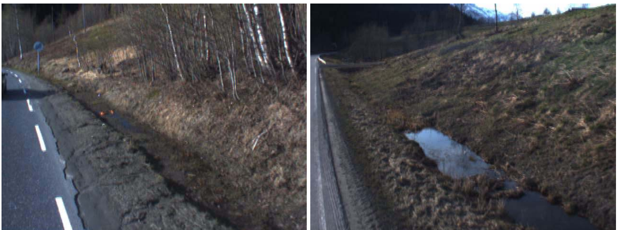
Figure 16: Water standing on the upper side of the slope, chainage left: 7370m, right: 34610m
