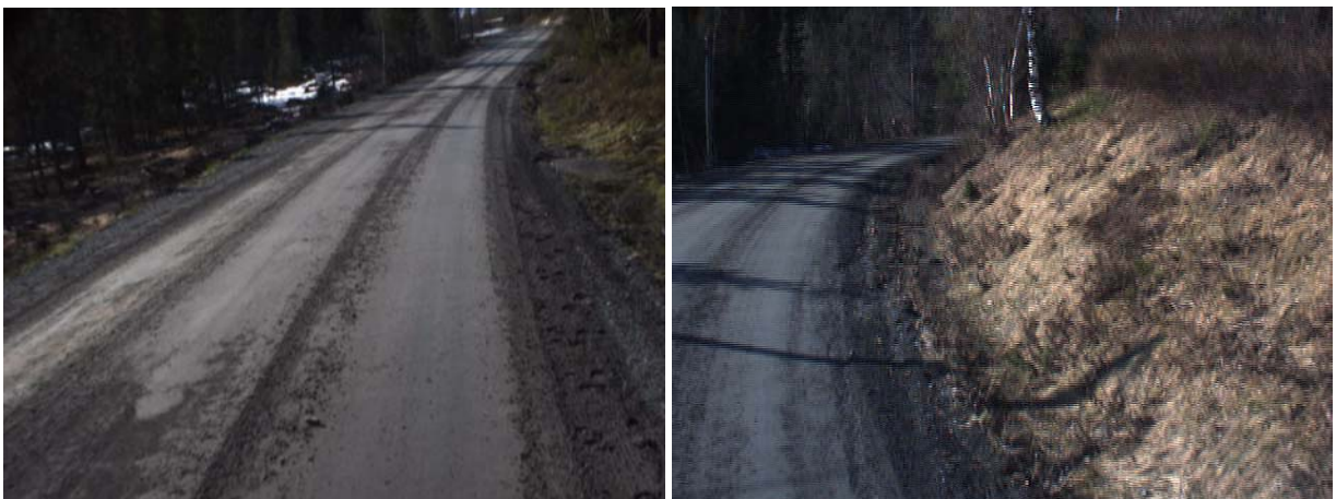
Figure 69: Drainage deficiencies on the upper side of the slope (Chainage 5430mm and 7600m)
