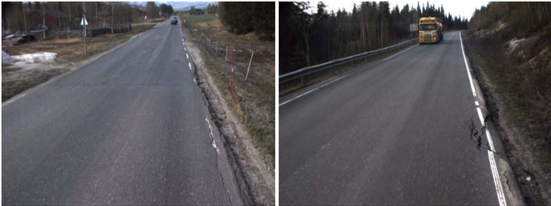
Figure 18: Erosion damages, chainage left: 1710m, right: 13635m
