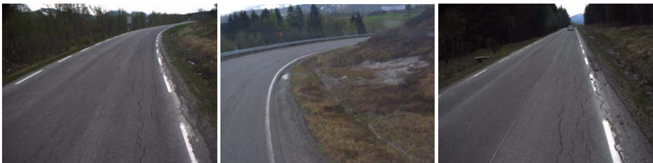
Figure 8: Examples of road sections with drainage Class 3 in Region Nord in Norway.
