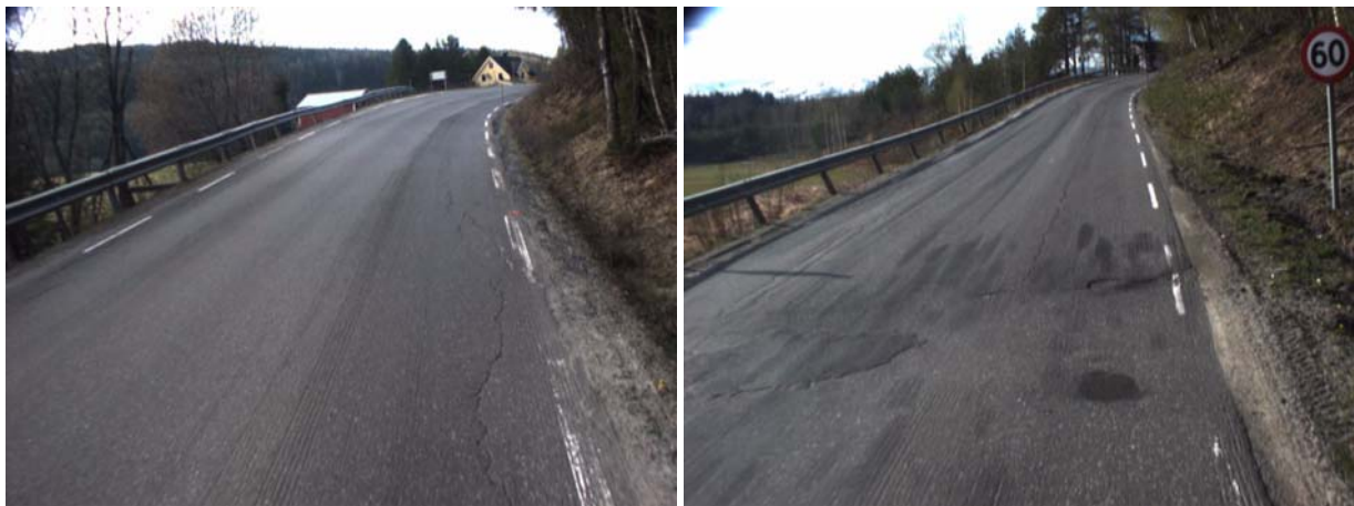
Figure 13: Little room for ditches on the upper side of the slope, chainage left: 995m, right: 5720m
