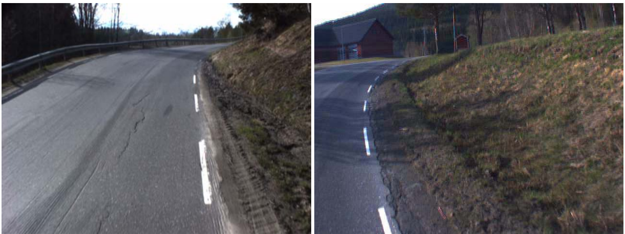
Figure 15: Drainage problems in a steep side sloping road profile, chainage left: 5650m, right: 7070m
