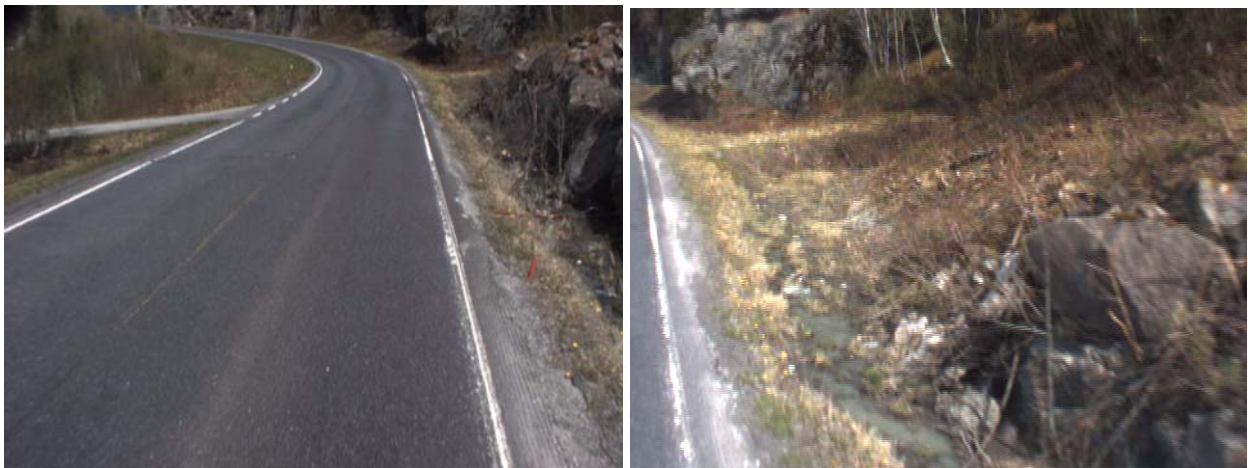
Figure 30: Example of rock cutting near the road. Left: general perspective at chainage 10400m and Right: detailed photo of clogged ditch at chainage 10440m.
