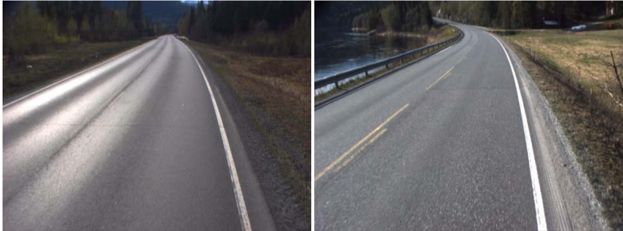
Figure 9: Two examples of verge Class 1, i.e. road sections without verges.
