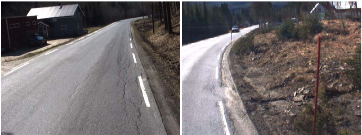
Figure 57: Unstable soil has filled the ditch and is blocking the water, chainage left: 3760m right: 5410m.
