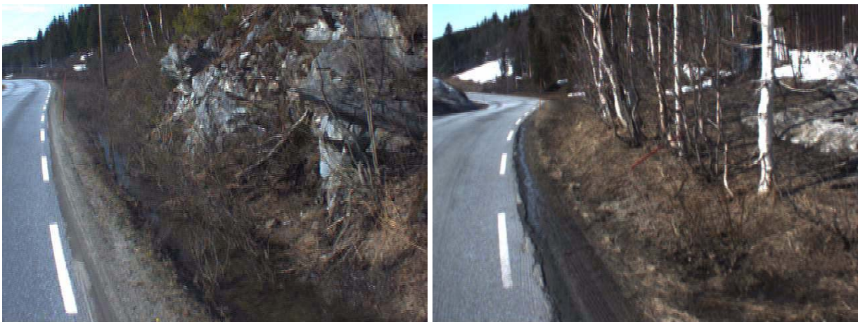
Figure 62: Inadequate drainage, chainage 4870m and 5060m.
