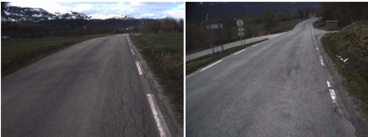
Figure 51: Shallow ditches, chainage left: 27870m, right: 28300m
