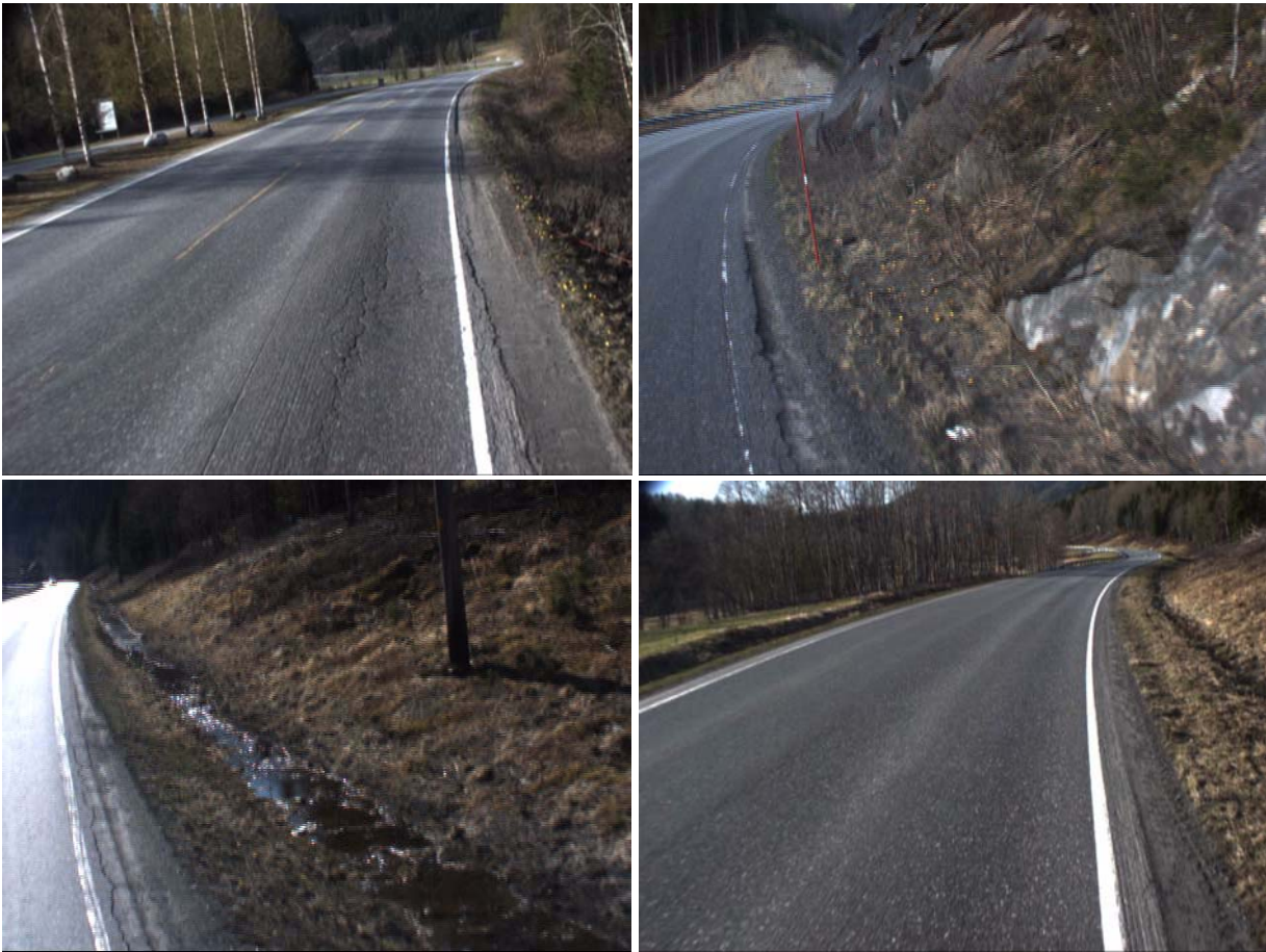
Figure 20: Ineffective drainage on the upper side of the side sloping road profile, chainages top left: 12350m, top right: 29330m, bottom left: 35270m, bottom right: 37220m
