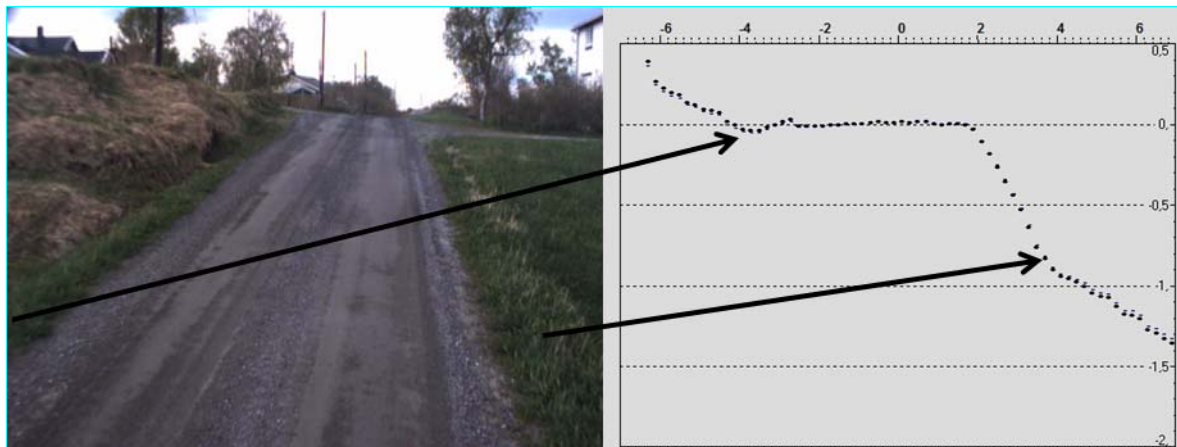
Figure 65: Inadequate ditch on the upper side of the slope, chainage 3060m.
