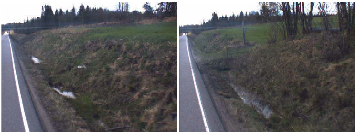
Figure 25: Left: Standing water in the ditch at chainage 6750m, Right: Partly blocked culvert in a private access road junction at 6800m
