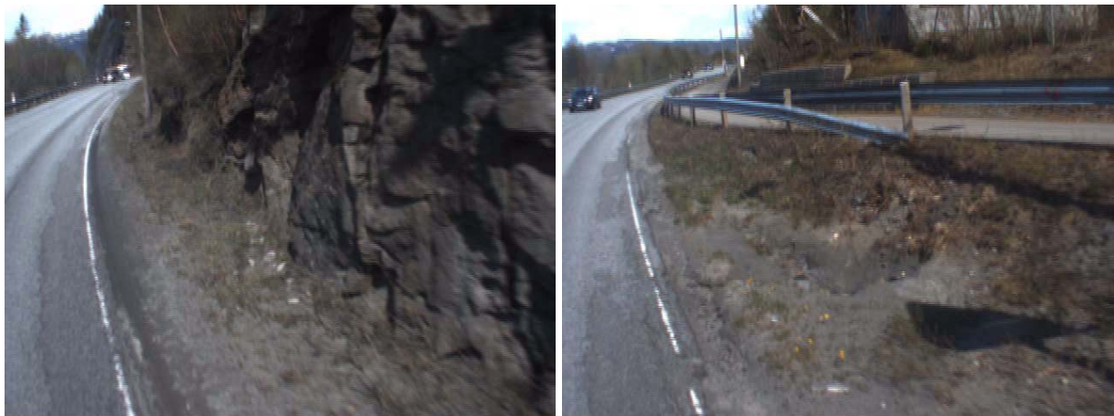
Figure 37: No ditches, chainage left: 2050m, right: 2530m
