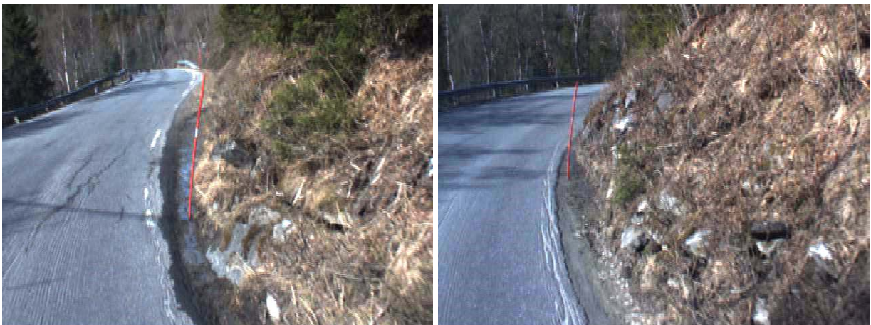
Figure 58: Steep side slope, not enough room for open ditch, chainage left: 6165m right: 6190m.
