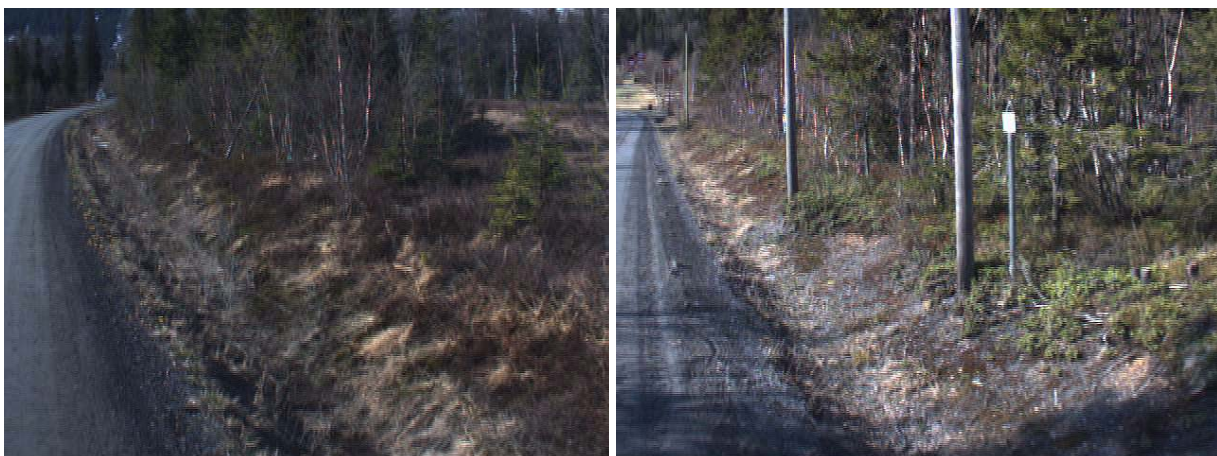
Figure 66: Shallow ditches at chainage 150m and 1000m.
