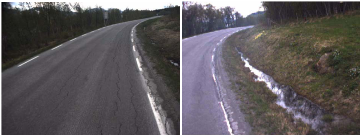
Figure 47: Typical drainage shortages for side sloping road profile, (chainage left: 1640m, right: 2900m)
