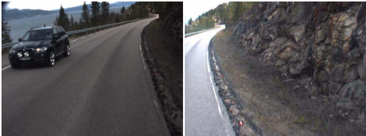
Figure 32: Examples of erosion damage; Right: Washout damage at chainage 2320m and Left: more detailed photo at chainage 2330m.
