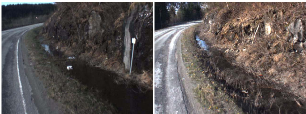
Figure 39: Severe drainage deficiencies, chainage left: 2500m, right: 5470m.
