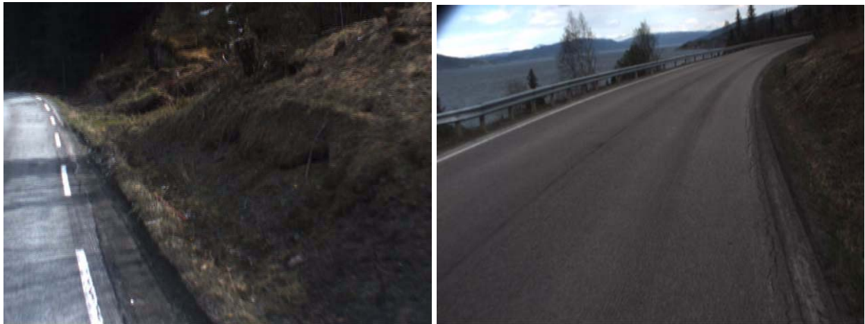
Figure 31: Examples of verge problems, Left: High verge at chainage 2970m, Right: Verge problem at 8130m chainage
