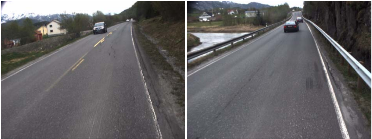
Figure 42: Left: Shallow ditch in side sloping road profile at chainage 19280m. Right: No room for a ditch between the cutting and guardrail at 21690m
