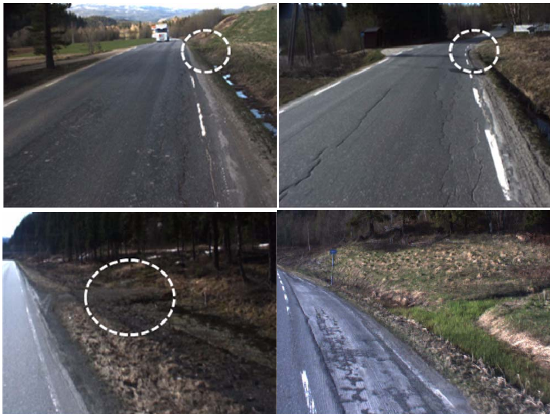
Figure 19: Examples of problems resulting mainly from private road access junctions and their culverts, chainages top left: 2250m, top right: 4300m, bottom left: 13495m. At chainage 32635m water is standing behind bus stop (bottom right).
