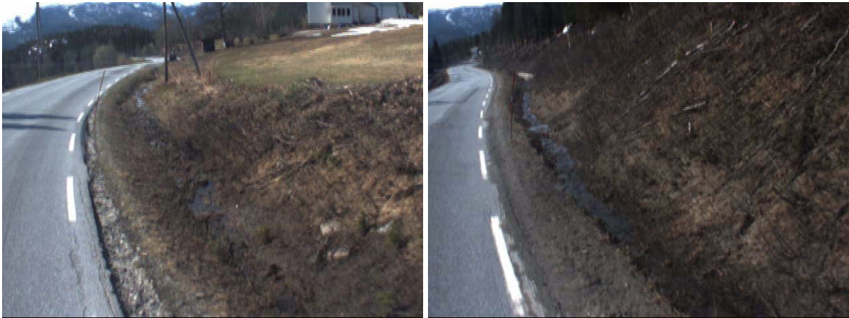
Figure 61: Shallow ditches and verge (also erosion damage on the left photo) were hindering the water flow, chainage left: 3700m, right: 4170m.
