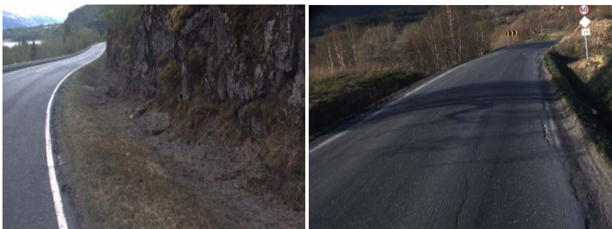
Figure 10: Examples of verge Class 2, roads with a verge. The effect of verges on the workings of the road drainage system varies greatly in different circumstances.
