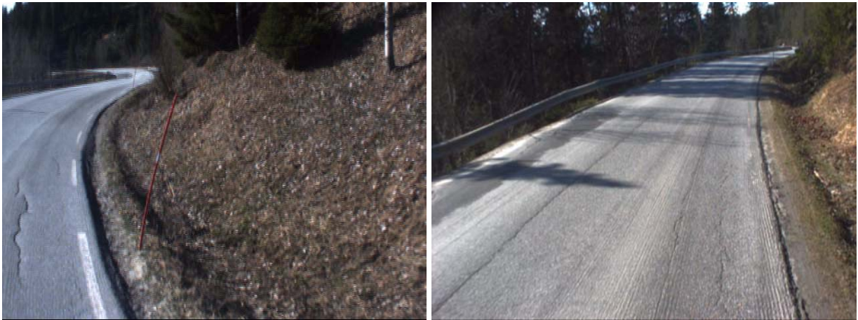
Figure 56: Inadequate ditch on the upper side of the slope, chainage left: 2380m, right: 3180m.
