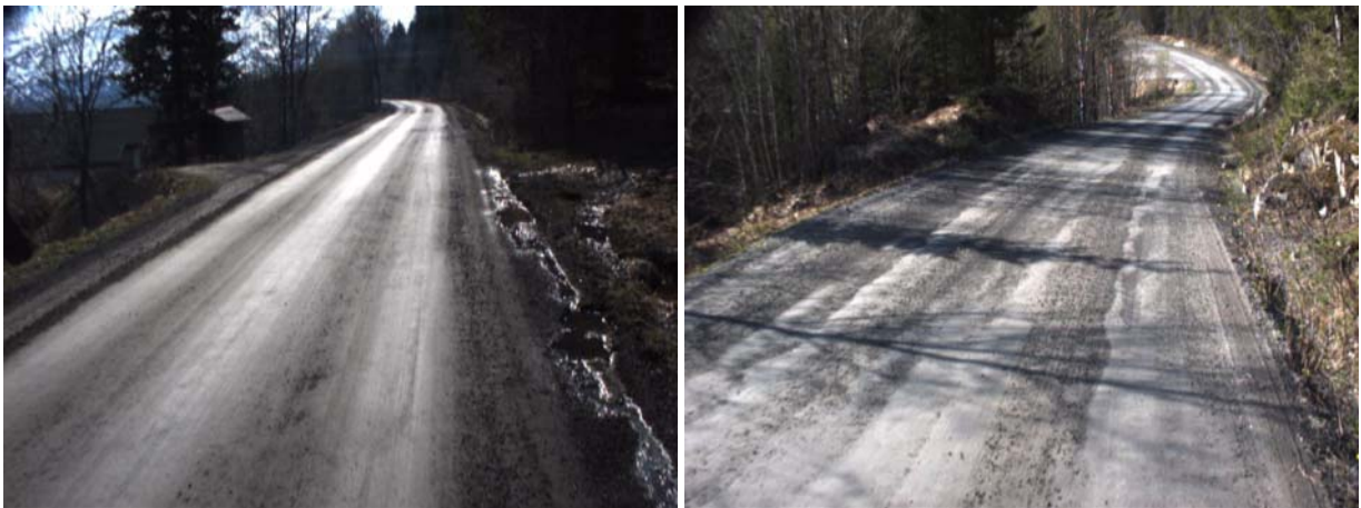
Figure 68: Drainage deficiencies on the upper side of the slope (Chainage 2130m and 4840m)
