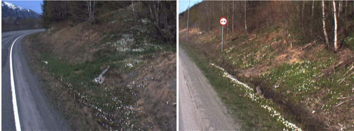
Figure 22: Inadequate drainage on the upper side of the side sloping ground (chainage 1600m, 1840m)
