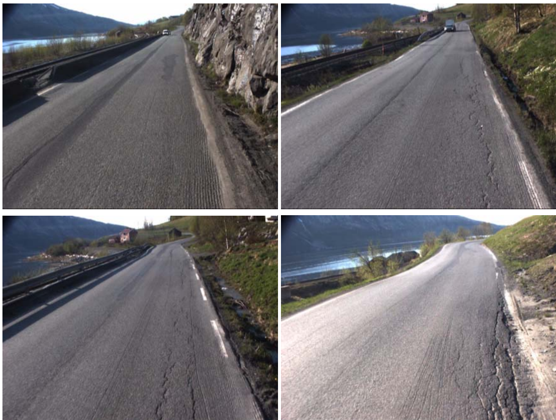
Figure 53: Drainage problems in steep side sloping road profile before the first tunnel, chainages shown from top left to bottom right: 850m, 1250m, 1330m and 1890m.
