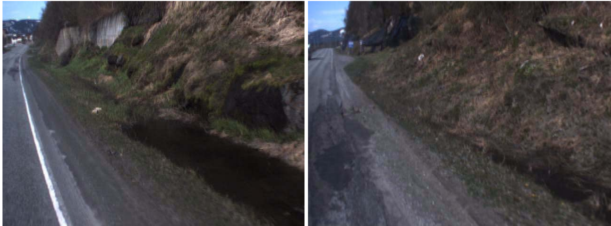
Figure 38: Partly filled ditch blocks the water flow at chainage 240m. Right: No ditch at 550m chainage.
