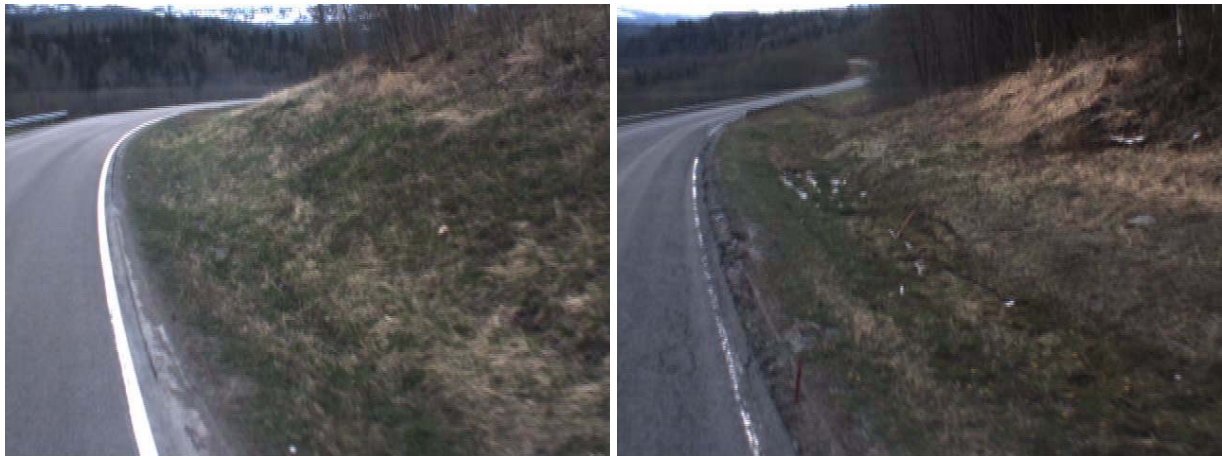
Figure 24: Problems with instability of the soil, also a verge problem chainage left: 1370m, right 2470m
