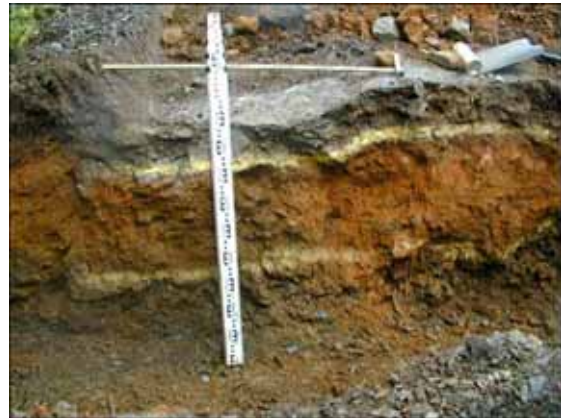
Figure 10. The pavement of Figures 2.8 & 2.9 seen in cross-section. (Layer boundaries picked out by spray-paint) (photo: courtesy W Tyrrell)
