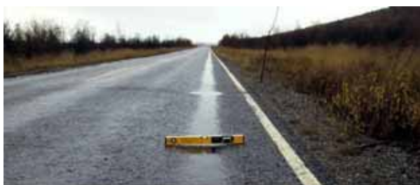
Figure 3. Water collecting in a wheel track of a thinly sealed pavement.
