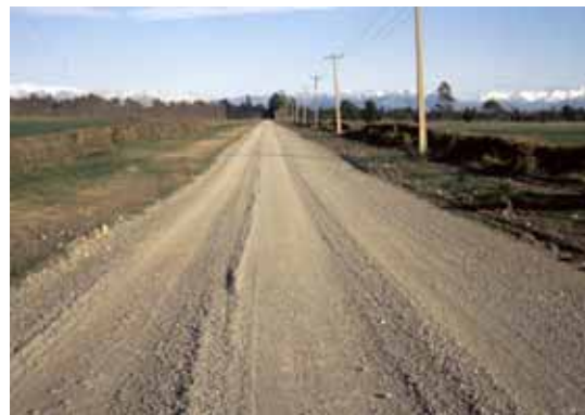
Figure 19. Partially crushed alluvial gravel in an unsealed pavement.
