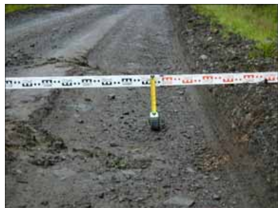
Figure 9. Close-up of rut in Scottish forest pavement. (photo: courtesy W Tyrrell)
