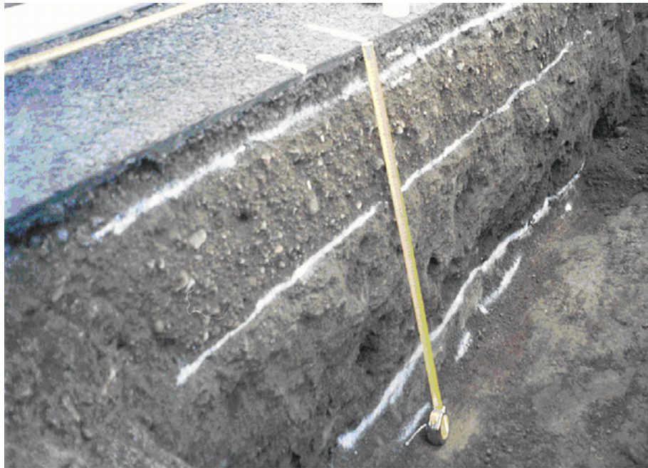
Figure 1. Cross sectional view of a thinly sealed pavement. (Layer boundaries picked out by spray paint) (photo: courtesy S Erlingsson)
