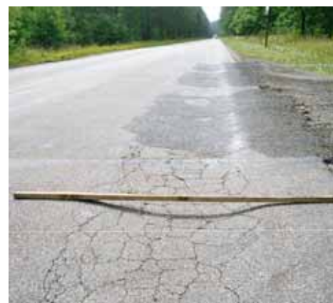
Figure 4. Rutting of a lower layers leads to distress in asphalt layers.
