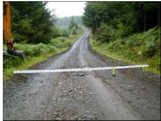
Figure 8. Scottish forest road exhibiting Mode 1 rutting. (photo: courtesy W Tyrrell)
