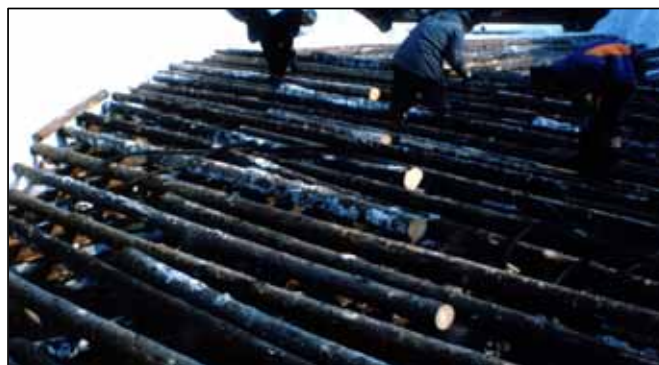
Figure 47. Photograph of an installation of a 2 layer pinned timber grillage.
