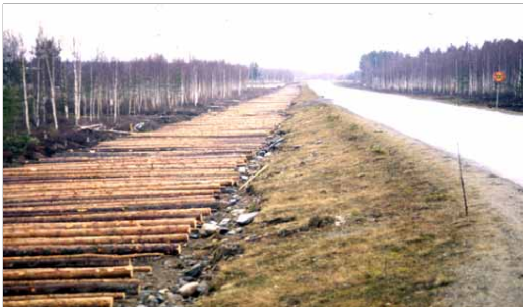
Figure 73. Widening of an existing road embankment with a timber grillage, Finland.
