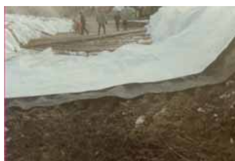
Geotextile, LECA and grillage
