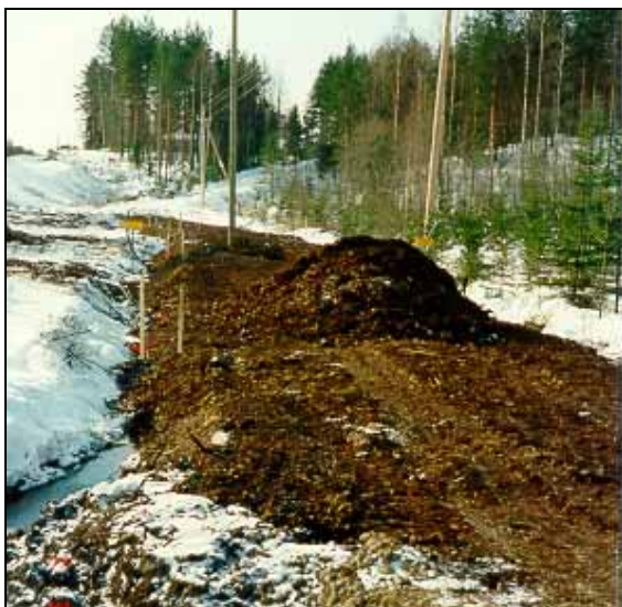
Chipped lightweight wood bark embankment core
