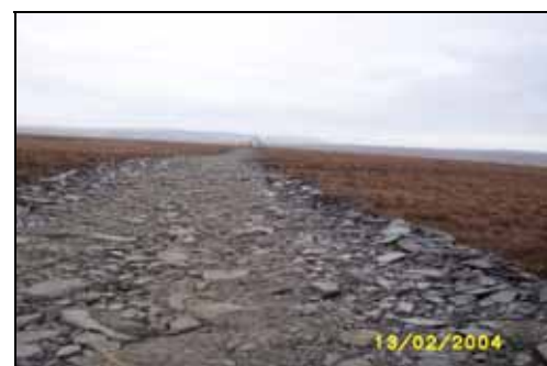
Photograph of rockfill roadway
