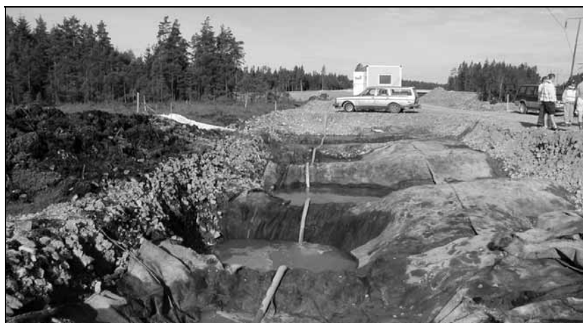
Photograph of exposed surface of the stabilised peat showing 'hills and valleys'
