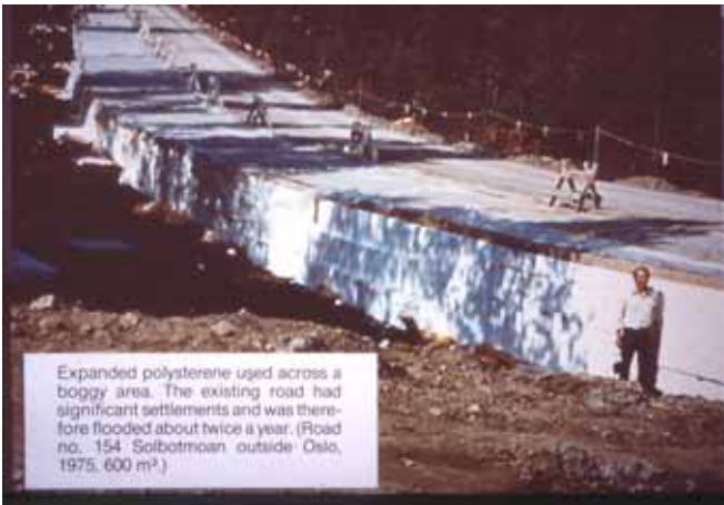
Photograph of the EPS embankment at
