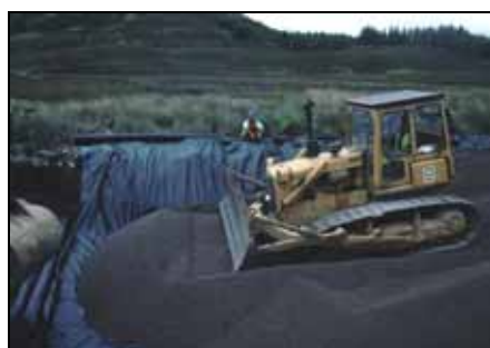
Placing of LECA lightweight fill
