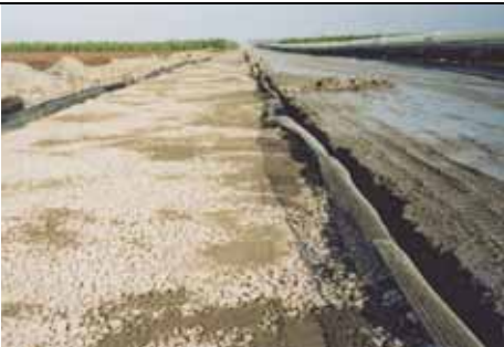
Geogrid backfilled with aggregate
