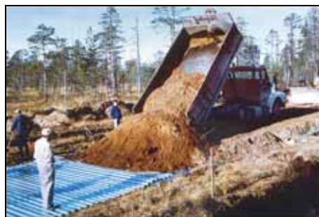
Figures 51. & 52. Photographs of road construction over peatland with “Geoprofile”
