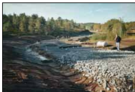
Photographs of the installation of geogrids and crushed rock on Road Fv-228, Fræna
