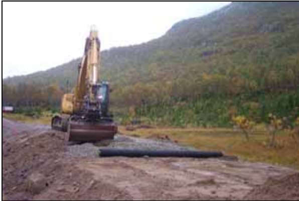
Rolling out geogrid on embankment and laying pavement
