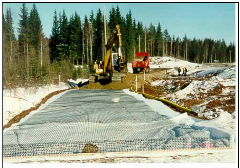
Installation of geotextile and geogrid on the wood chip embankment
