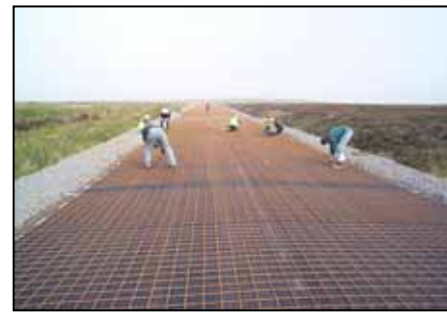
Steel mesh installation
