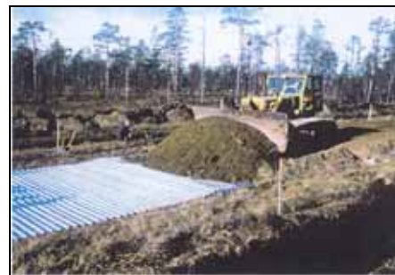
Figures 51. & 52. Photographs of road construction over peatland with “Geoprofile”
