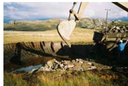
Typical site photographs of peat excavation on strategic roads within The Highland Council area
