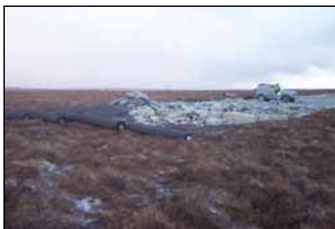
Photograph of rockfill being placed
