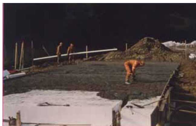
Casting of concrete slab and integral ribs
