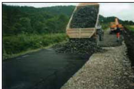
Photographs of the installation of geogrids and crushed rock on Road Fv-228, Fræna
