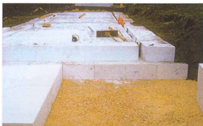
Placing of EPS blocks on sawdust layer
