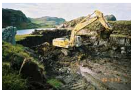
Typical site photographs of peat excavation on strategic roads within The Highland Council area
