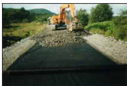
Photographs of the installation of geogrids and crushed rock on Road Fv-228, Fræna
