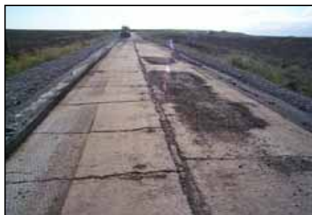
70 year old concrete slab surface exposed
