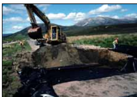
Excavation of existing embankment
