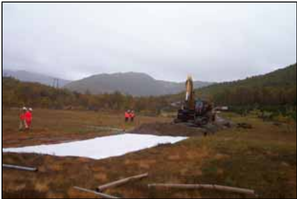
Filling over geotextile placed on bog surface
