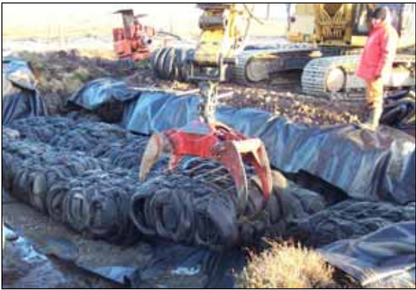
Installation of tyre bales in embankment
