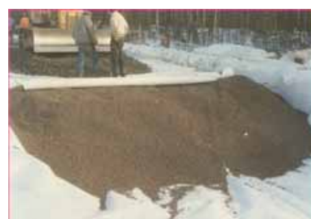
Geotextile and lightweight filling
