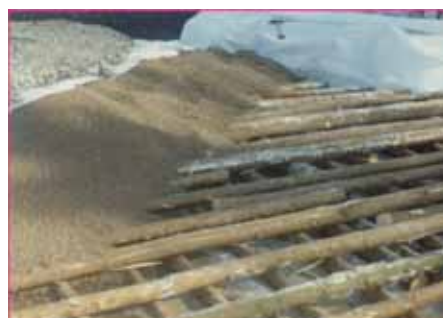
Geotextile, LECA and grillage
