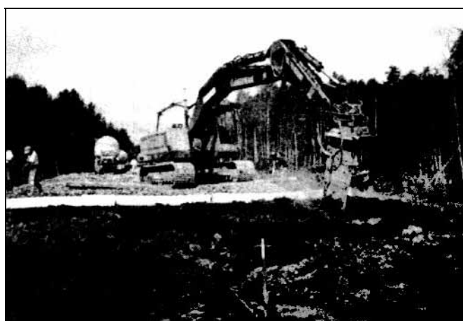
Photograph of mass stabilisation works
