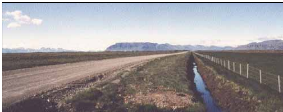
Figure 37. Icelandic road over peat showing advance ditches.
