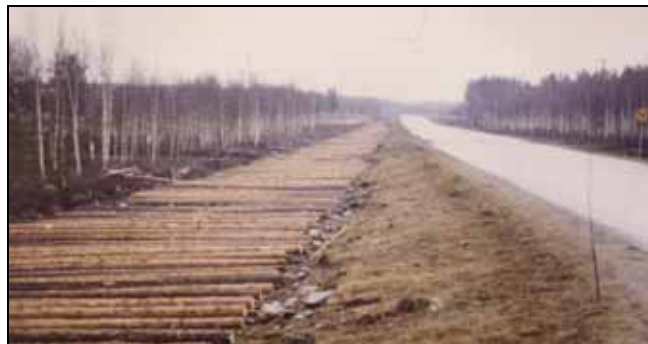
Figure 46. Photograph of a simple timber corduroy platform in a road widening.
